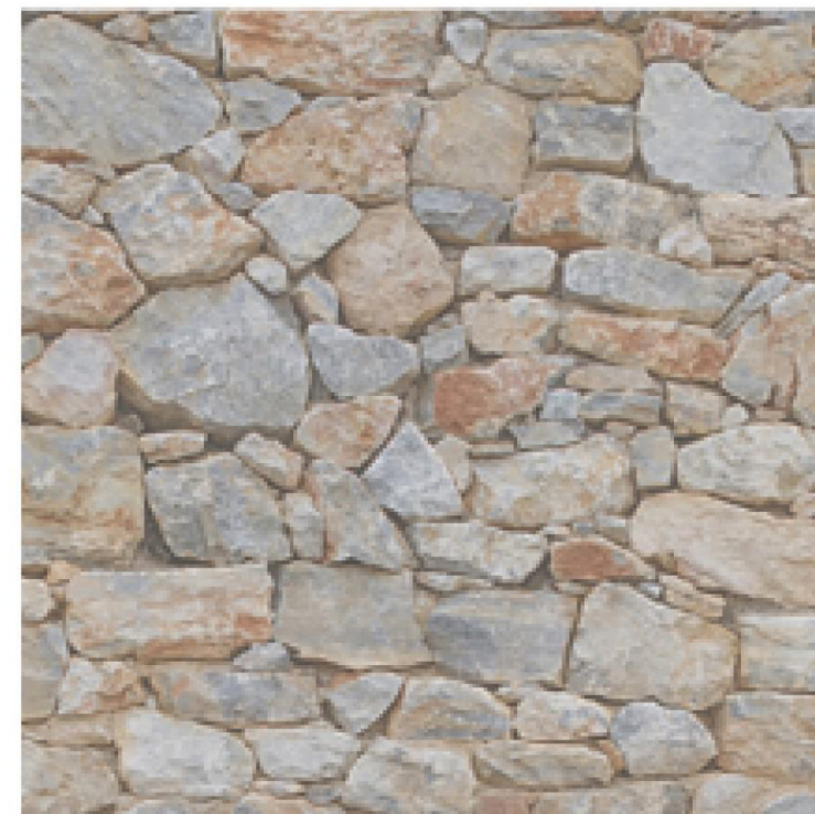
STONE EXTERIOR WALL
