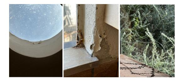
**4. Door/ Window Hardware Repair:** Window hardware needs to be restored/repaired to maintain weather resistance and comfortability. The wooden doors are worn and weathered. General maintenance and repairs are needed to avoid further deterioration.
