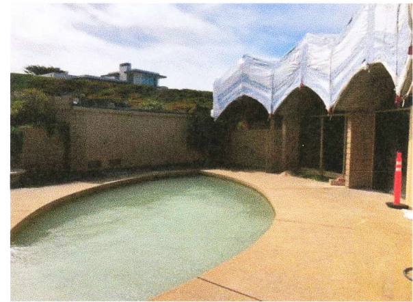
COURTYARD VIEW – GARAGE NORTH WALL
