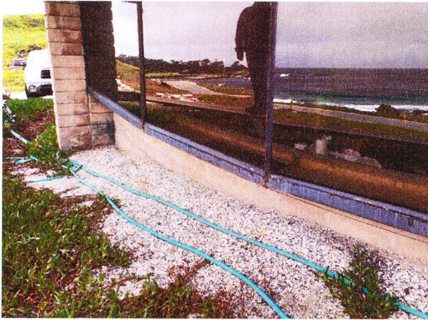
Painted steel sill of projected window wall
