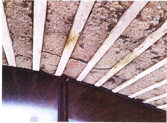
Cracked concrete at window wall due to water intrusion and rebar corrosion
