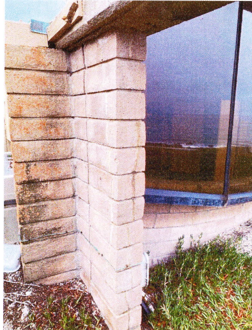
Northern most column and remnants of original trellis at roof edge
