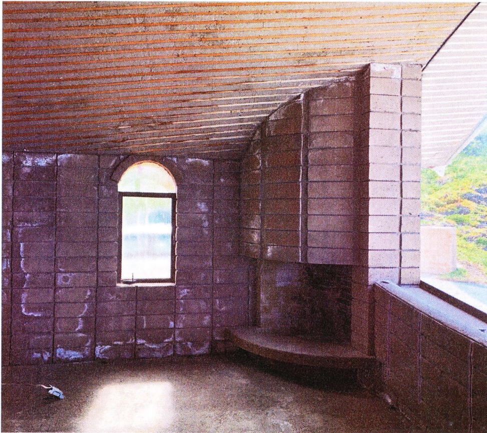
Interior view of south exterior wall at Primary Bedroom. Water intrusion from damaged roof edge, and chimney. Proposed replacement trellis at end walls would capture roof water run off in a new gutter to reduce water sheeting over the roof edge down the wall face.
