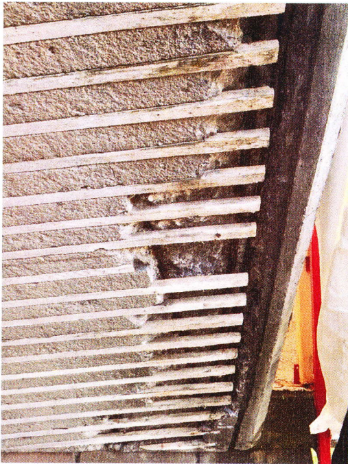
Removal of patched concrete to expose extent of corrosion of rebar. Exploration uncovered corrosion from roof edge to window line was consistent at each roof segment.
