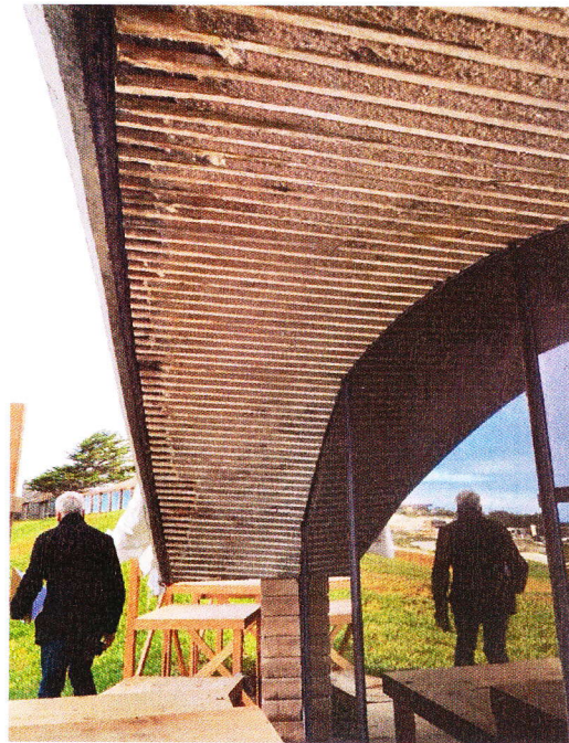
Removal of patched concrete to expose extent of corrosion of rebar. Exploration uncovered corrosion from roof edge to window line was consistent at each roof segment.
