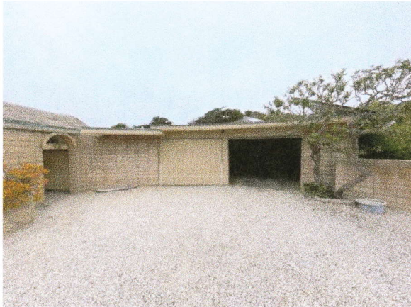
GARAGE FROM PARKING AREA
