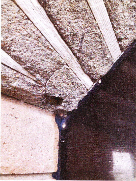
Cracked concrete at window wall due to water intrusion and rebar corrosion
