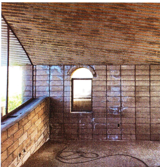
Interior view of south exterior wall at Primary Bedroom. Water intrusion from damaged roof edge, and chimney. Proposed replacement trellis at end walls would capture roof water run off in a new gutter to reduce water sheeting over the roof edge down the wall face.
