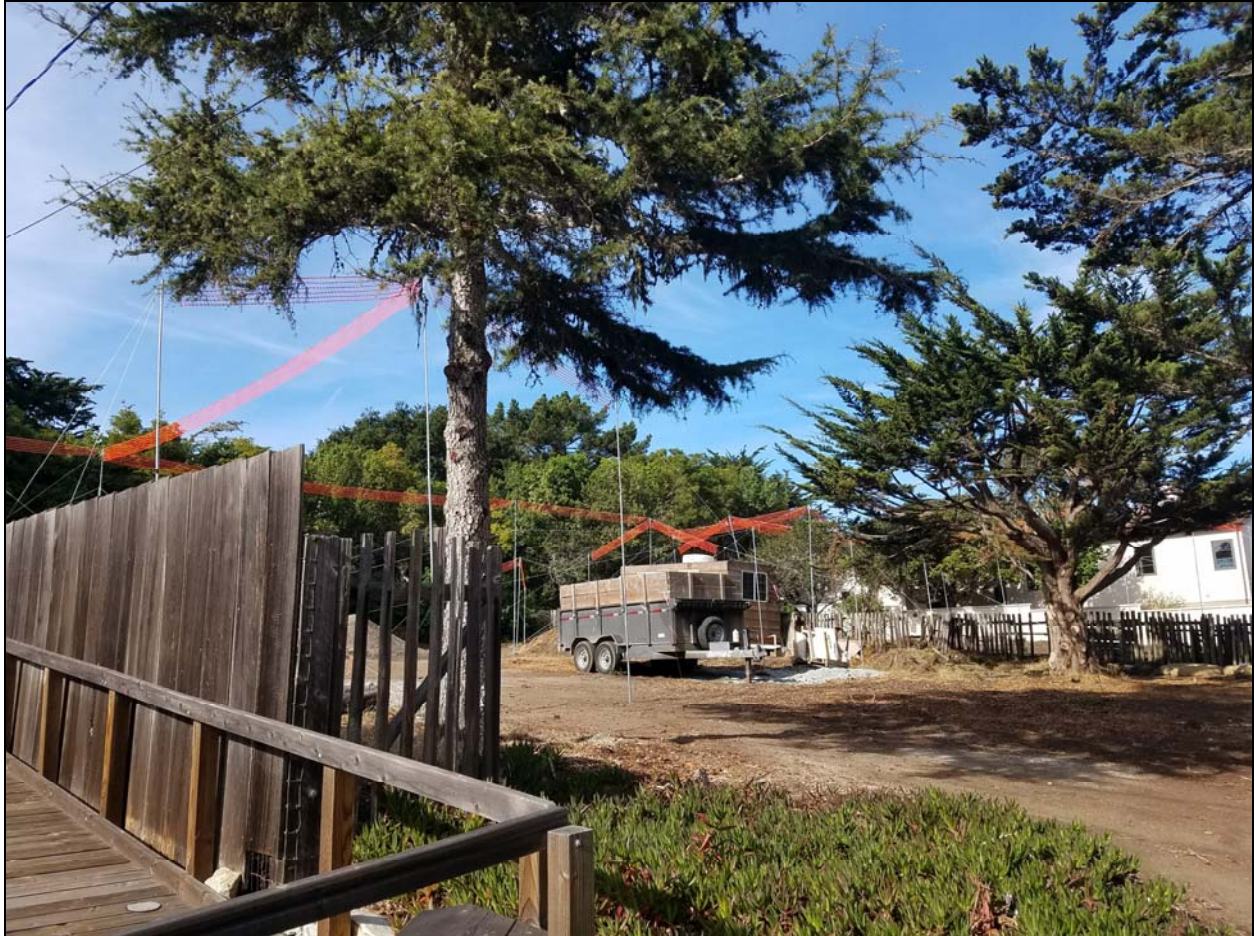
Figure 15b – Site Visit Photos: Staking and Flagging at 26346 Valley View Avenue
