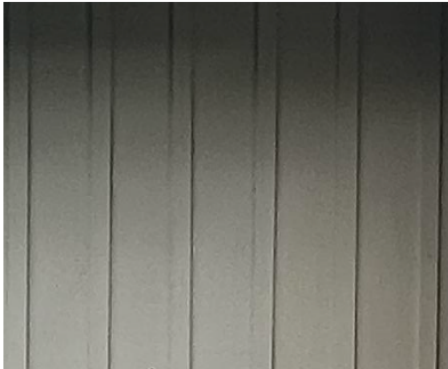
BOARD & BATTENS SIDING NEW SIDING TO MATCH EXISTING B&B MATERIAL: WOOD FINISH: PAINT
