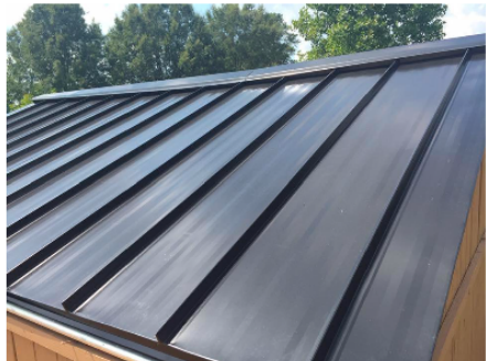
METAL ROOF MANUFACTURER: TAYLOR METAL PRODUCTS FINISH: CHARCOAL GRAY SRI-25 GAUGE: 24 LVR: 12
