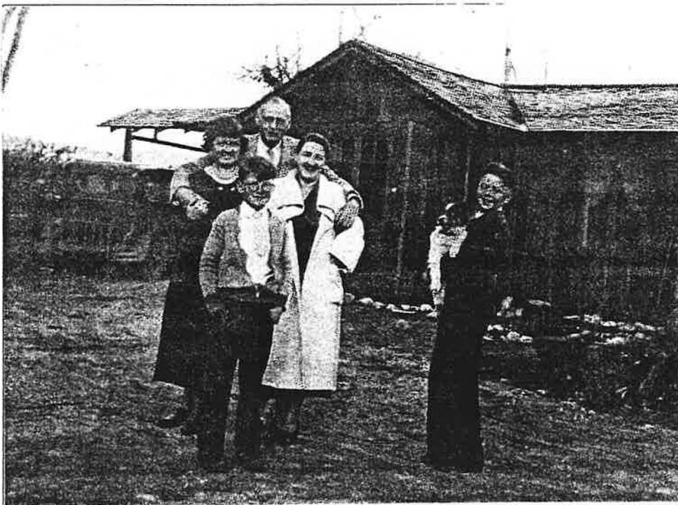
Description of Photo: (View, date, accession#) Looking NE at the w/facing facade of cabin #11, Orville Jones, 1934, Kathleen Jones Col., Phoenix, AZ
