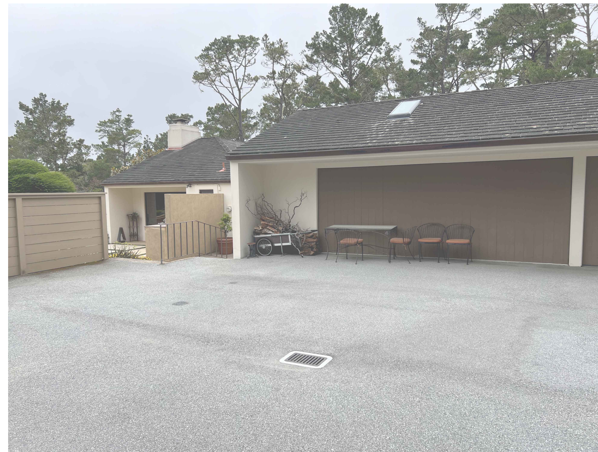
2 EXISTING PHOTOGRAPH LOOKING WEST AT EXISTING GARAGE & EXTERIOR SIDE OF KITCHEN TO BE RENOVATED WITH NEW ADDITION
