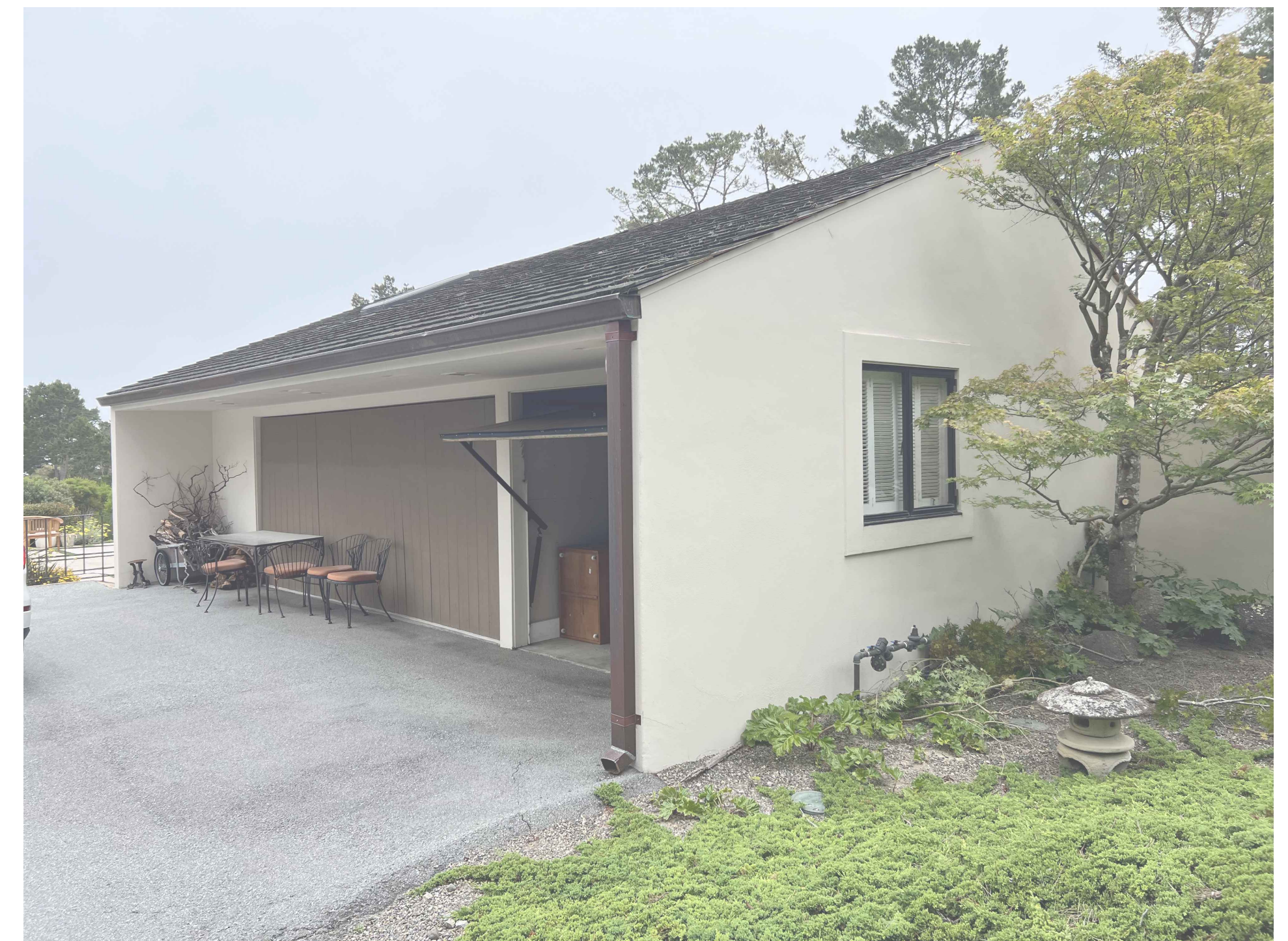
1 EXISTING PHOTOGRAPH LOOKING WEST AT EXISTING GARAGE TO BE RENOVATED
