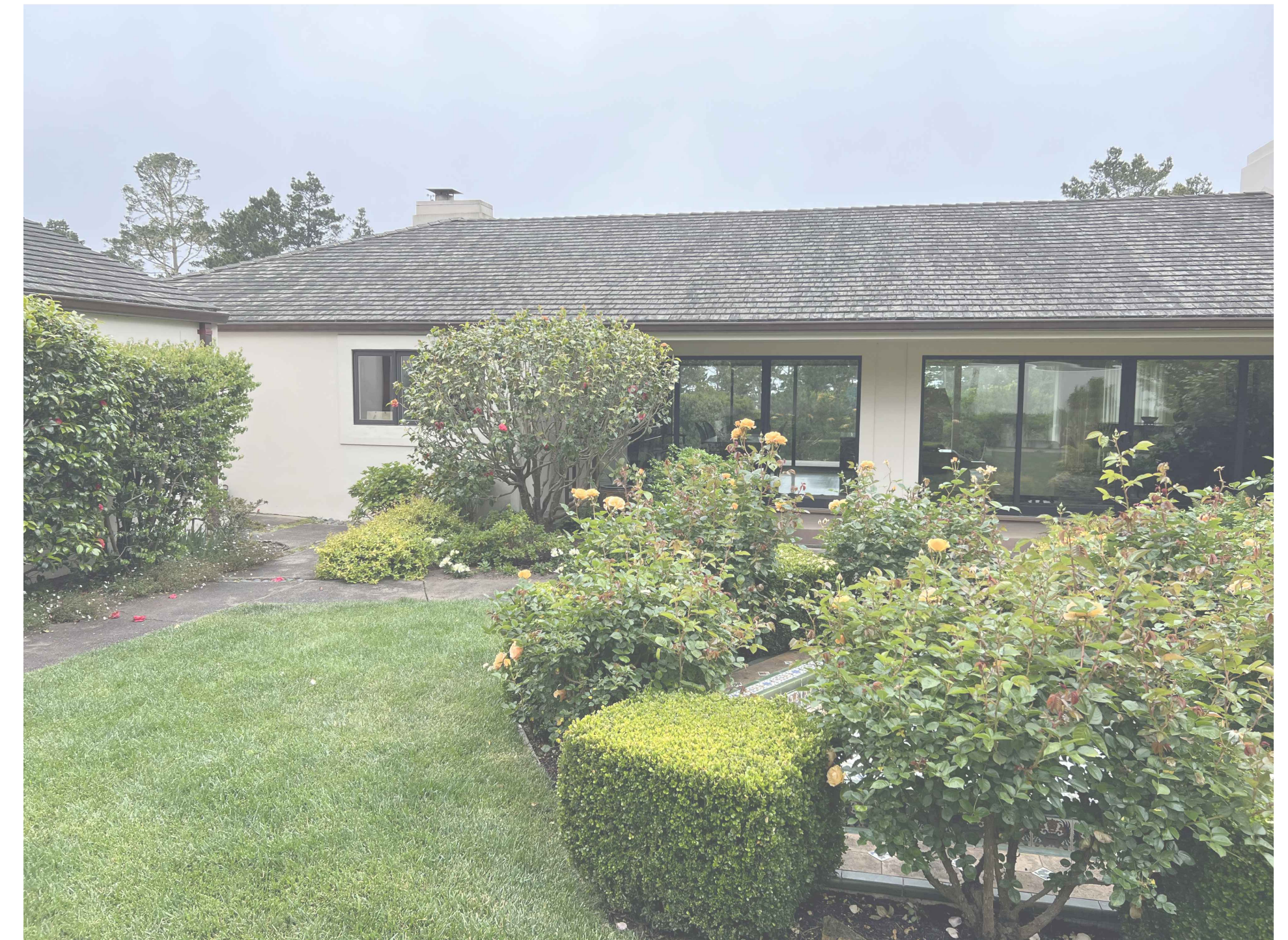
4 EXISTING PHOTOGRAPH LOOKING SOUTHWEST AT EXISTING RESIDENCE; AREA OF ROOF TO BE RENOVATED AT NEW ADDITION ON THE UPPER LEFT
