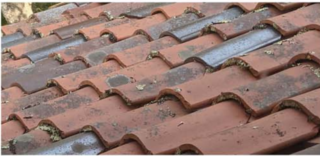
TERRACOTTA CLAY TILE ROOF - MATCH EXISTING
