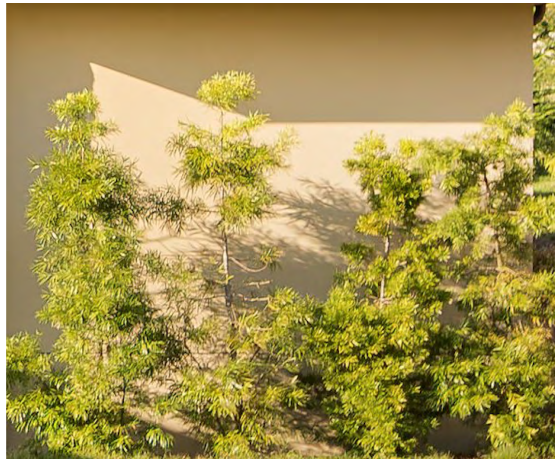
EXTERIOR PAINTED STUCCO
