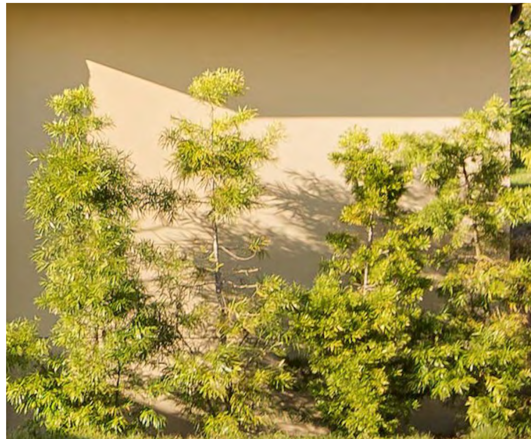
EXTERIOR PAINTED STUCCO
