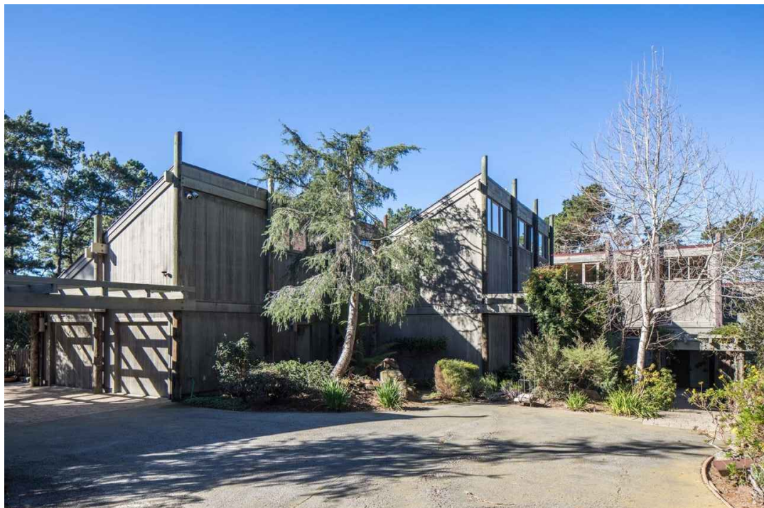
FRONT OF HOUSE & GARAGE
