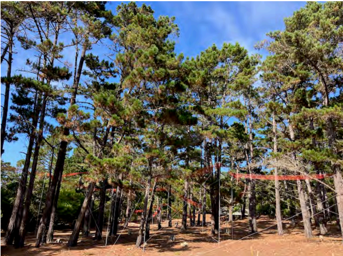
Figure 4. Another view of proposed homesite from Deer Path road. This parcel is dominated by mature and aging Monterey pines, several of which are in poor and declining physiological health and structural condition.
