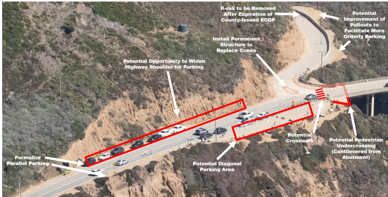
Figure 1: North End of Bridge and Old Coast Road
