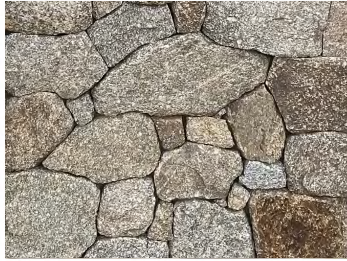
LOCALLY SOURCED, UNCOURSED RANDOM ASHLAR STONE WALLS
