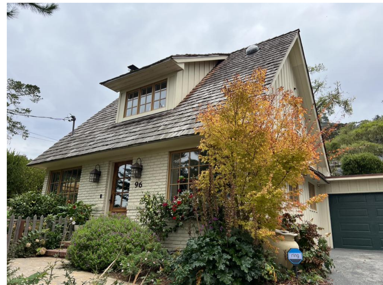
MAIN ENTRY (WEST ELEVATION)
