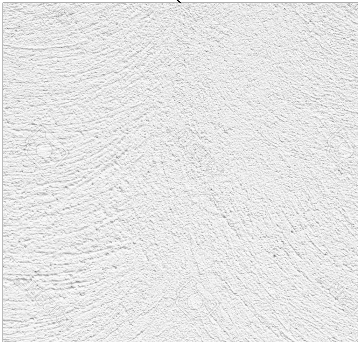
PAINTED CEMENT PLASTER AT FLAT ROOF ELEMENTS
