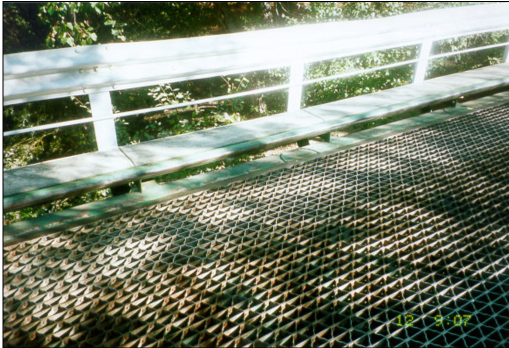
VIEW OF DECK STEEL GRATING
