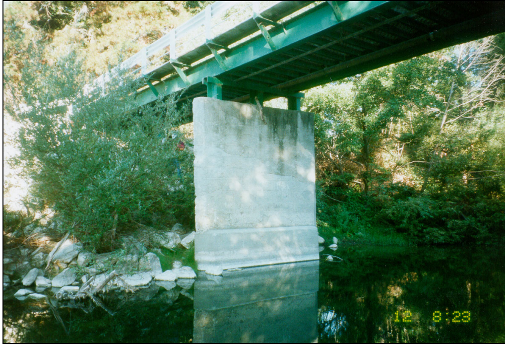
VIEW OF CONCRETE PIER LOOKING SOUTH
