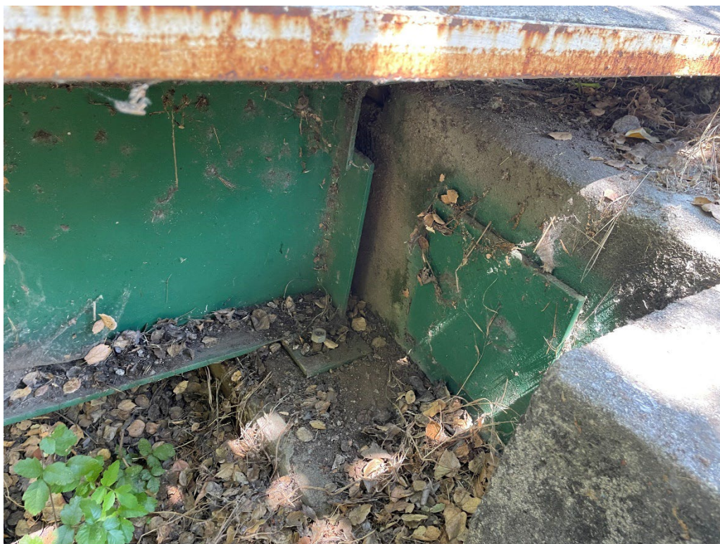
Photo 10: Anchor bolts at east abutment
