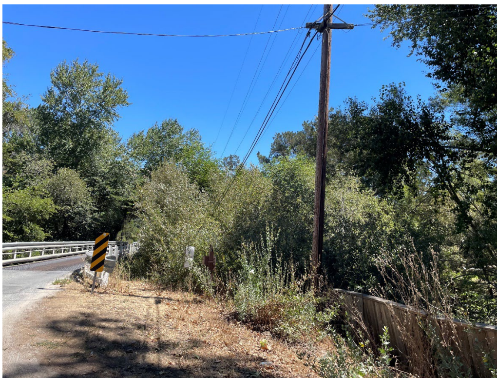
Photo 3: Looking east. New bridge will be widened to the south.
