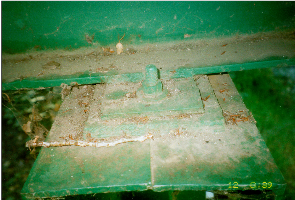
VIEW OF ANCHOR BOLTS UNDER GIRDER
