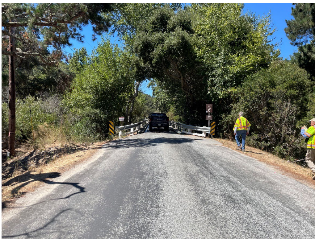
Photo 1: Looking west. Note narrow bridge width and lack of sidewalks.
