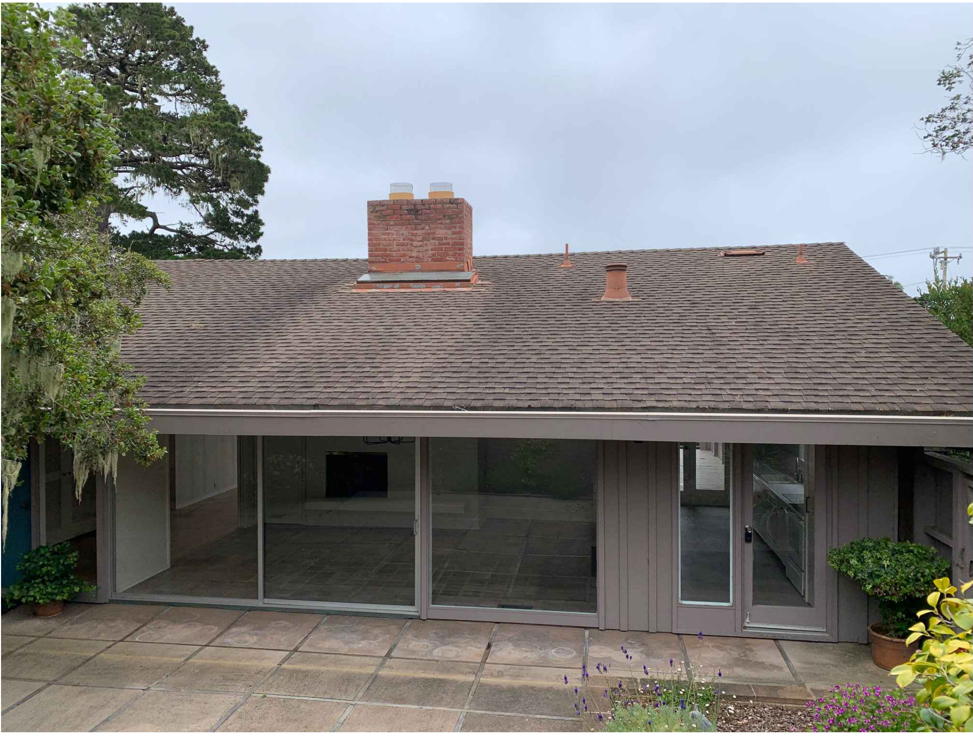
VIEW SOUTH AT DRIVEWAY
