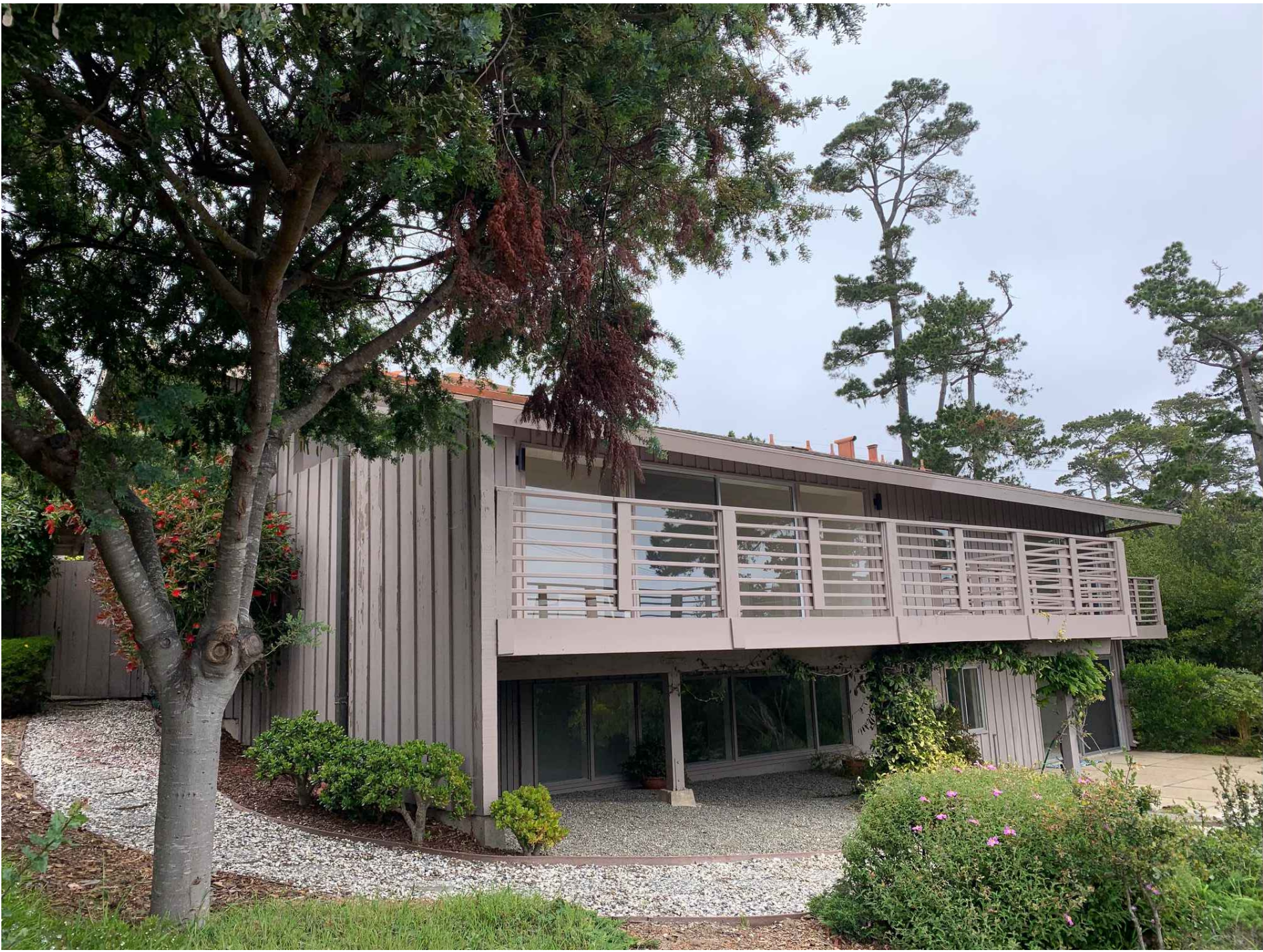
VIEW AT NORTHEAST CORNER
