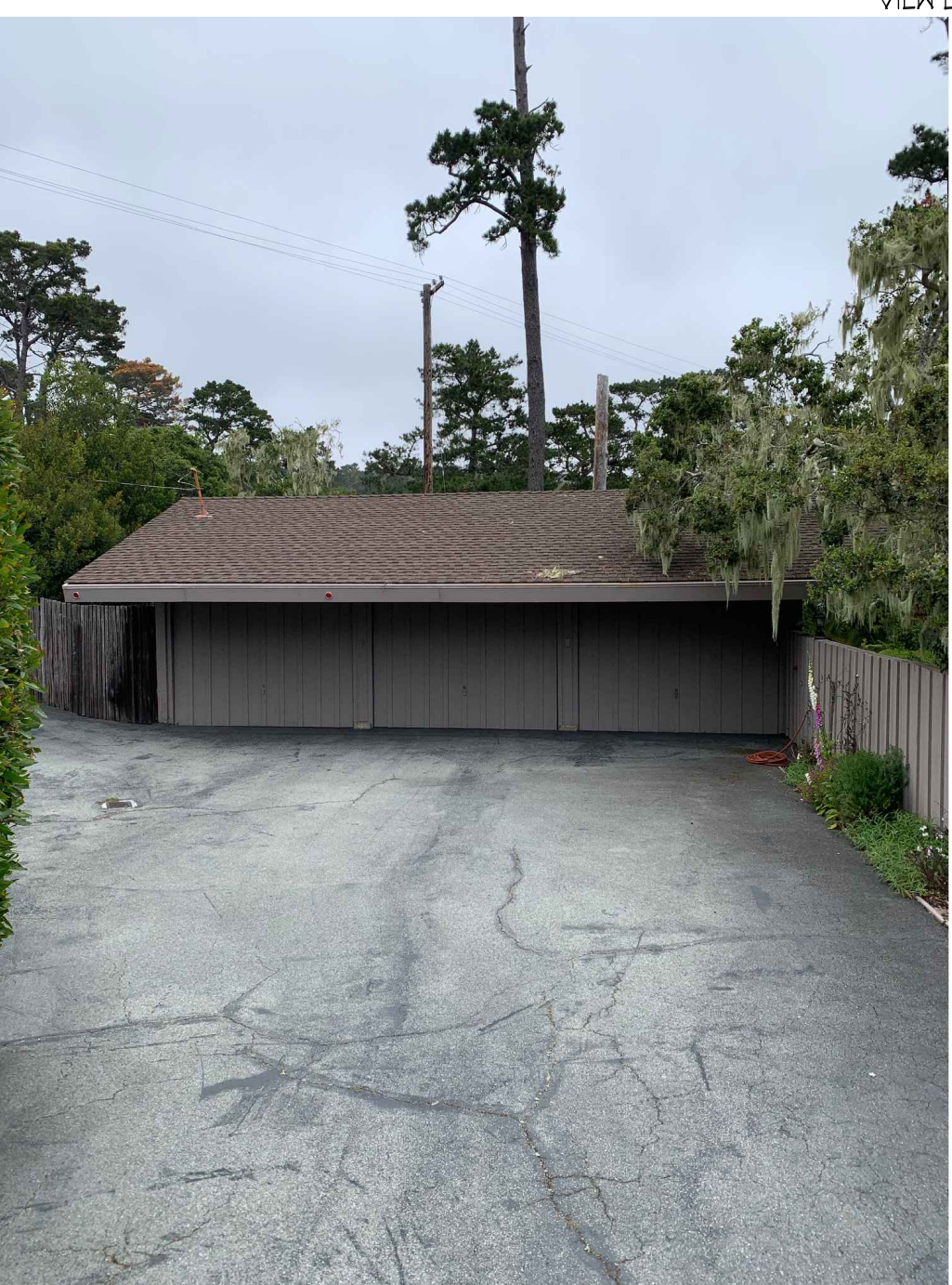
VIEW LOOKING EAST AT DRIVEWAY
