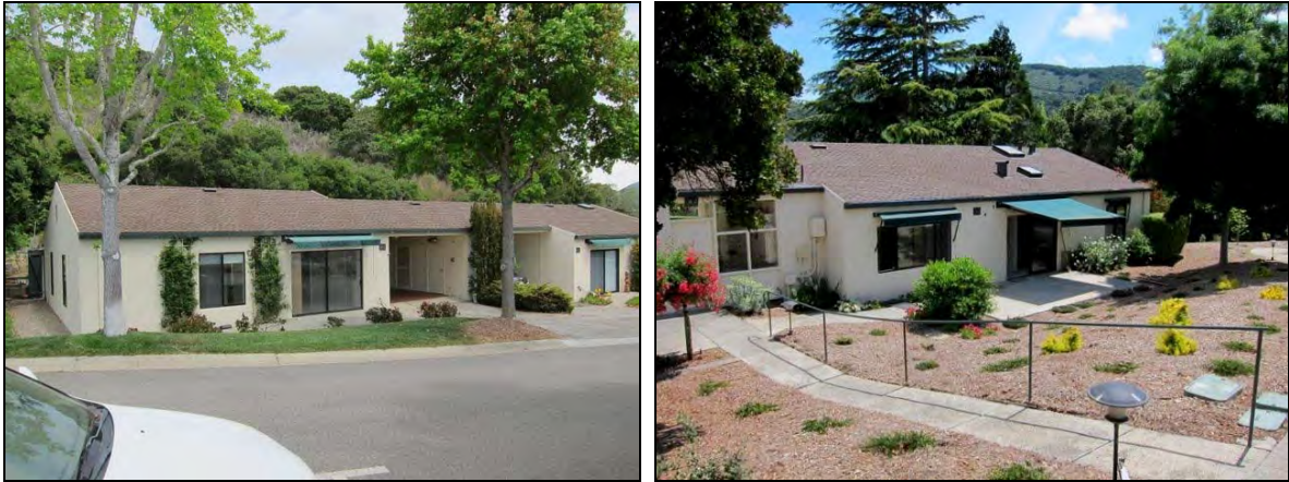
Figures 8 and 9. Typical front and rear elevations of Building Type D. Right image shows window added to rear wall as part of typical carport conversion.
