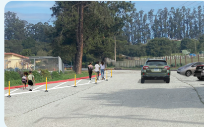
Pedestrian pathway in driveway of Echo Valley Elementary School
