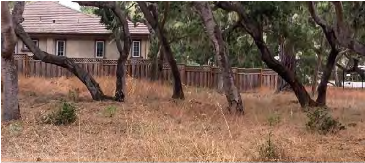
Figure 5: Wooden fences are a fire risk, because they can trap embers and ignite during a wildfire event, leading the fire directly to the home.
