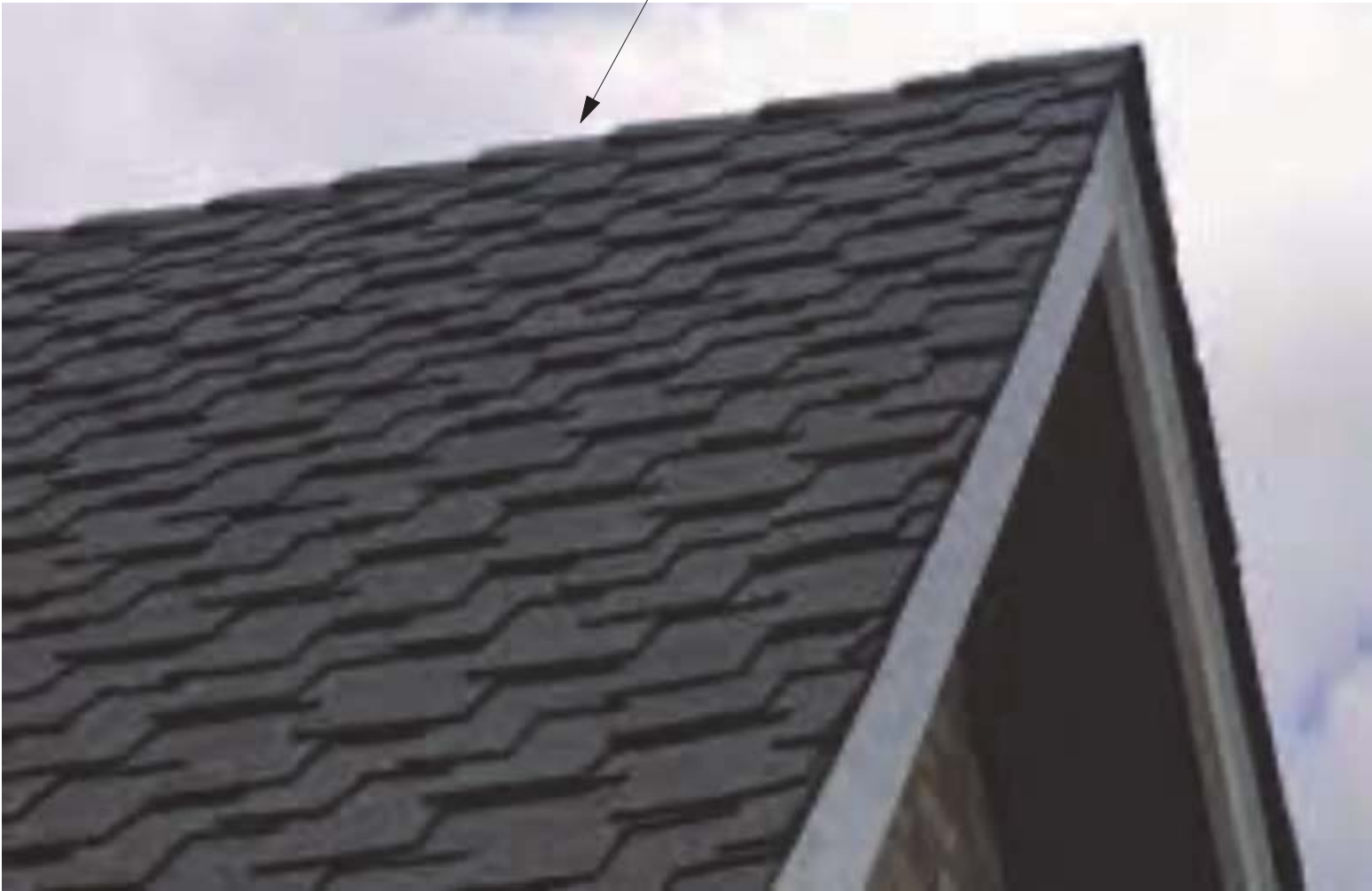
50 YR. COMPOSITION ROOFING (COLOR: CHARCOAL)
