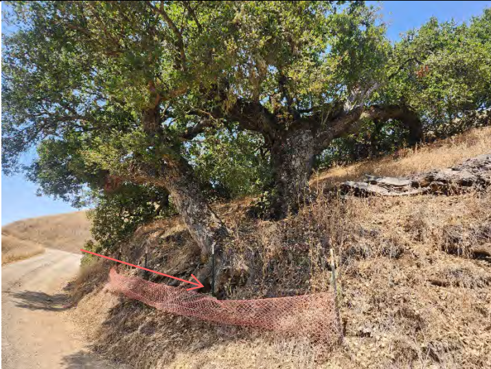
Tree #13 (left); Recommended for removal, soil eroding under tree. Tree #36 (right); Within grading limits for retaining wall footprint.
