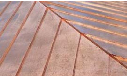
COPPER STANDING SEAM ROOM
