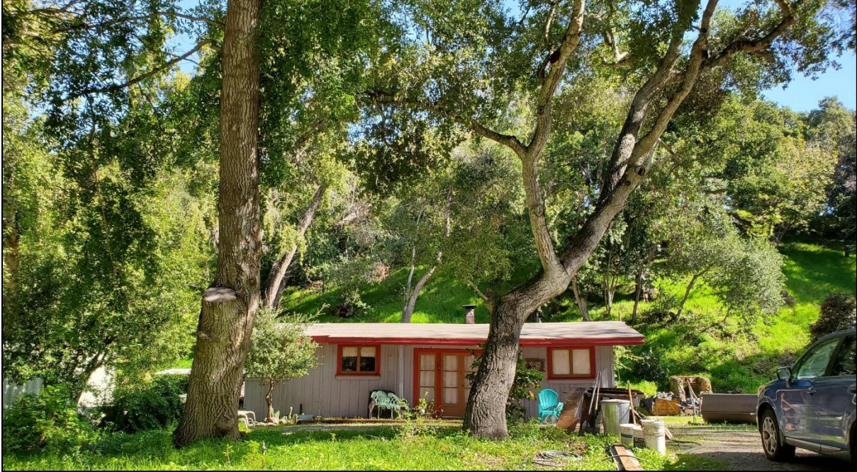
Figure 6 – Cabin to be replaced.
