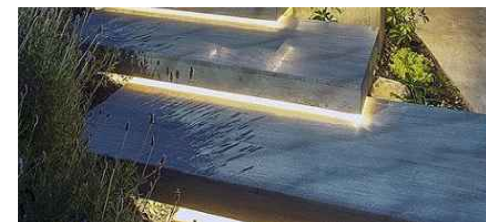
EXTERIOR STEPS WITH UNDERLIGHTING
