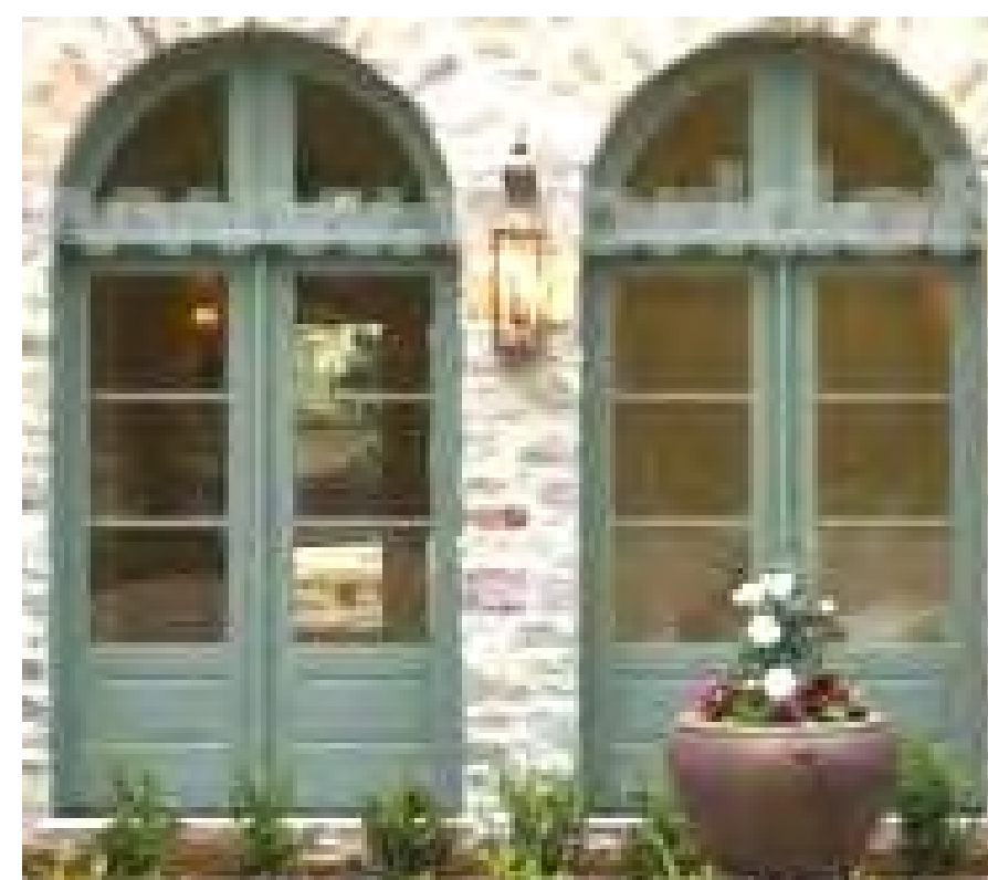
5 WINDOW FRAM/TRIM ALUMINUM-CLAD WOOD, PAINTED SAGE GREEN
