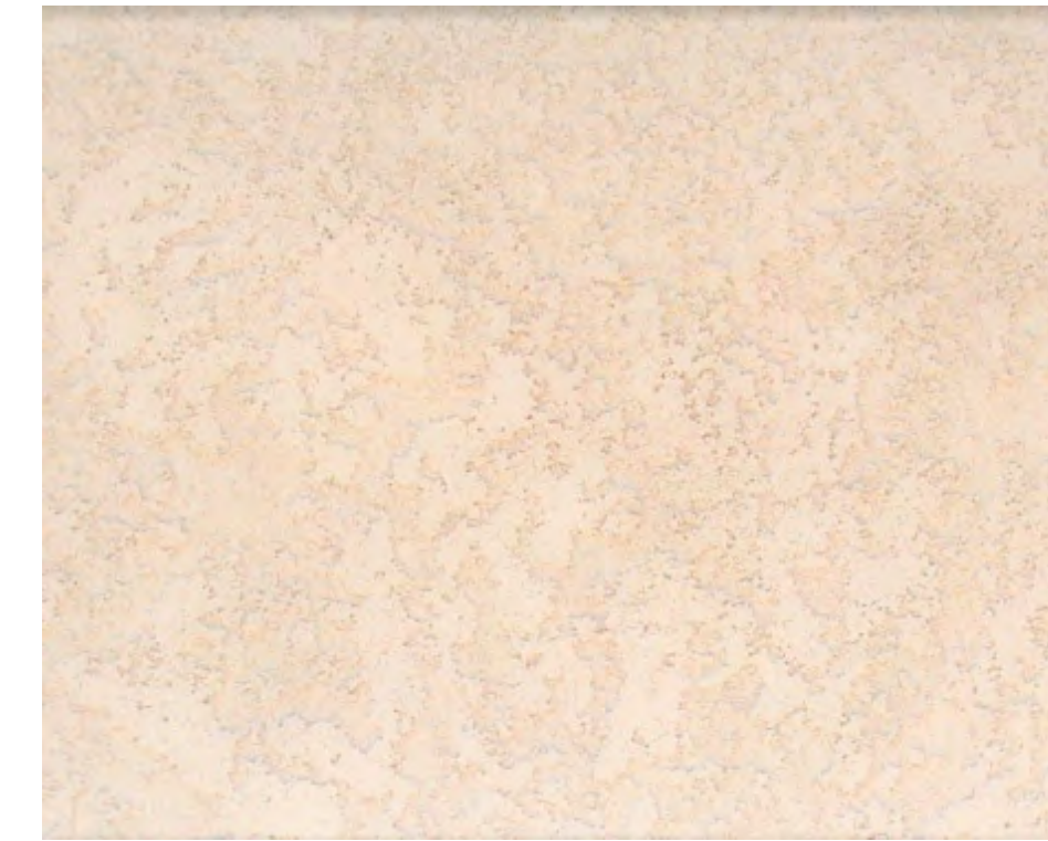
3 STUCCO SMOOTH FINISH, PAINTED LIGHT YELLOW
