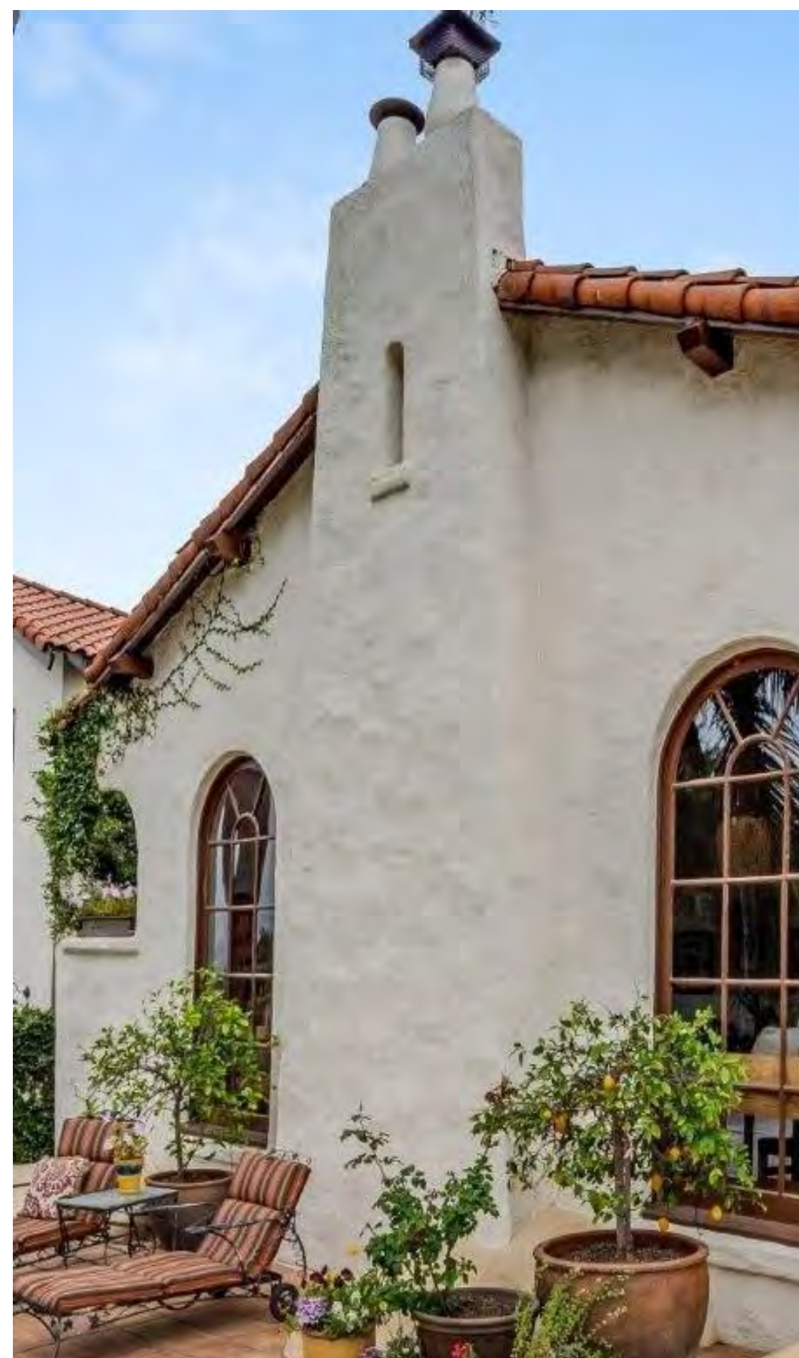
13 CHIMNEY, STUCCO SMOOTH FINISH, PAINTED LIGHT YELLOW
