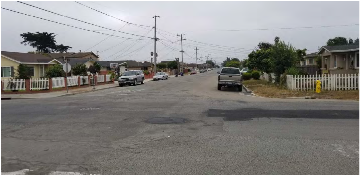
Mead St/Pomber St Intersection looking southeast
