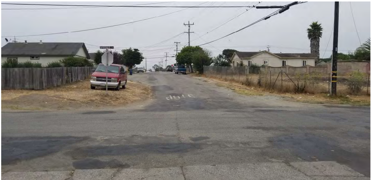
Speegle St/Seymour St Intersection looking southeast
