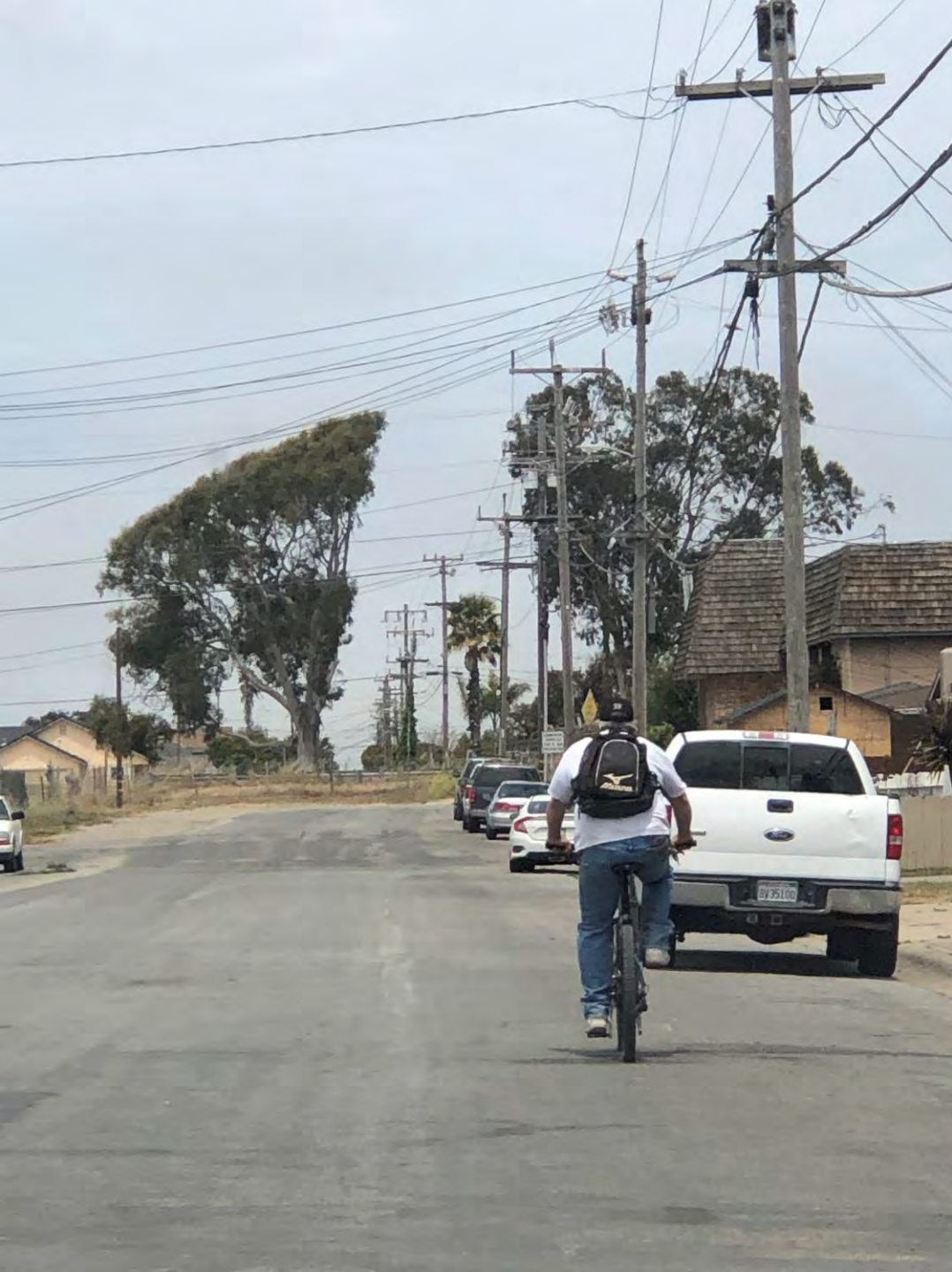
Left: Seymour Street: Proposed Improvements include curb, gutter, sidewalks, ADA ramps and Class III Bike Lanes.
