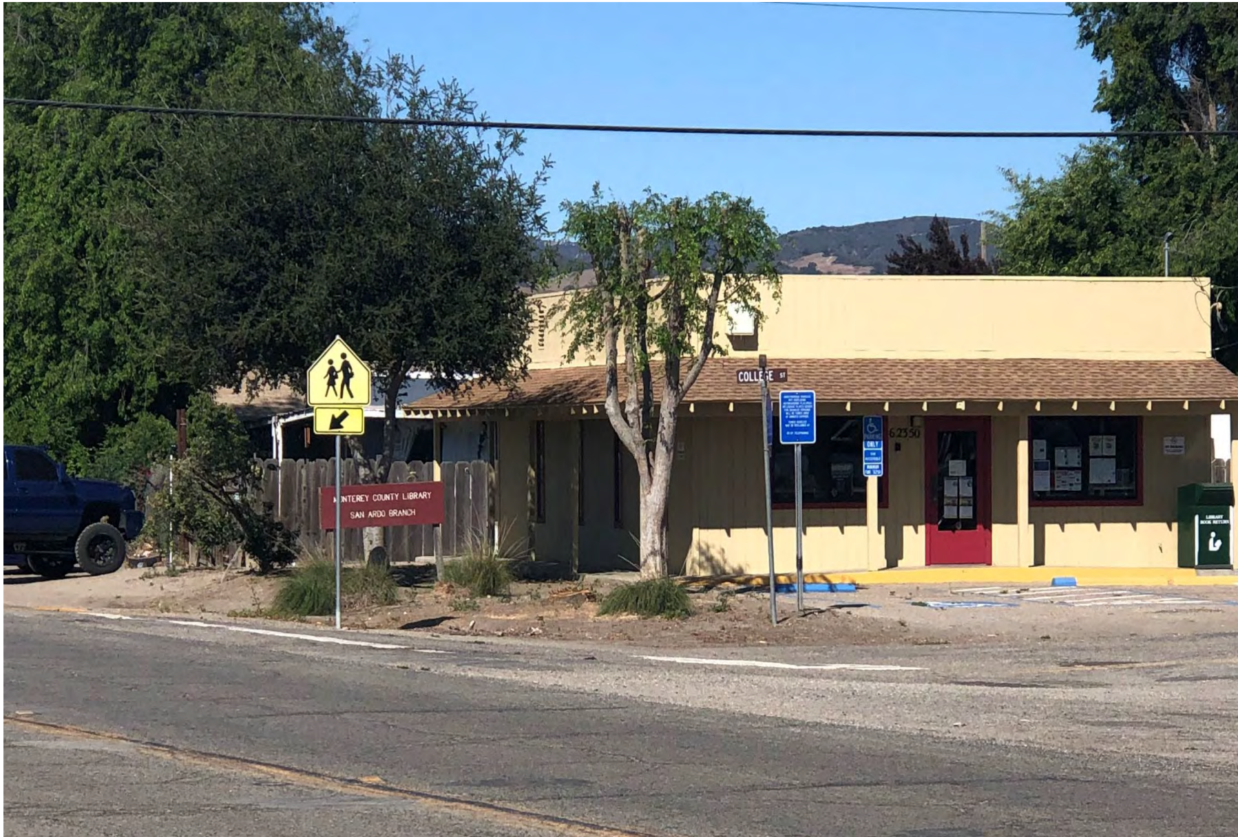
Library at Intersection of Cattlemen Road and College Street- Proposed improvements to this intersection include crosswalk, curb and gutter along College Street in front of the Library.
