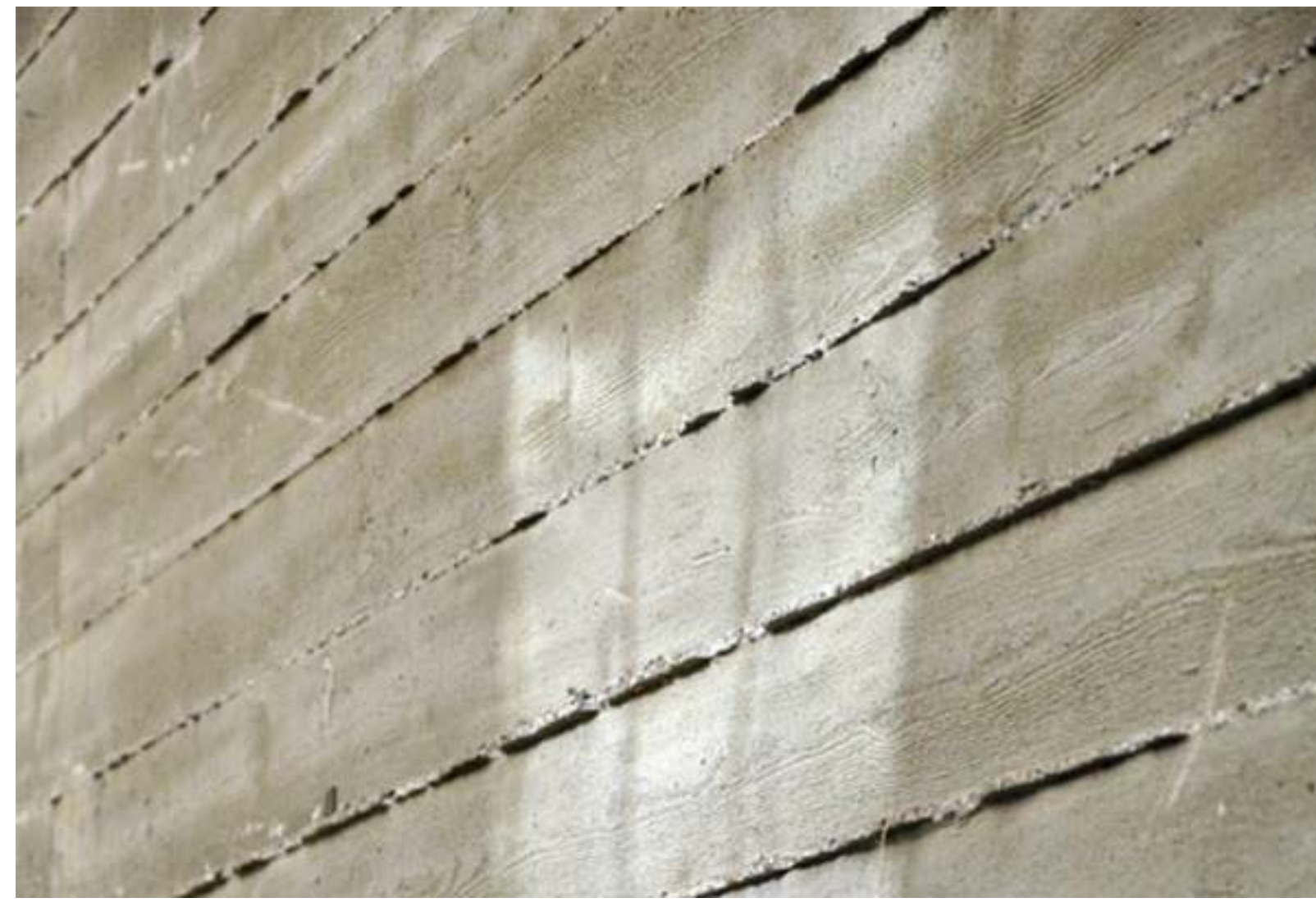
BOARD FORMED CONCRETE WALLS
