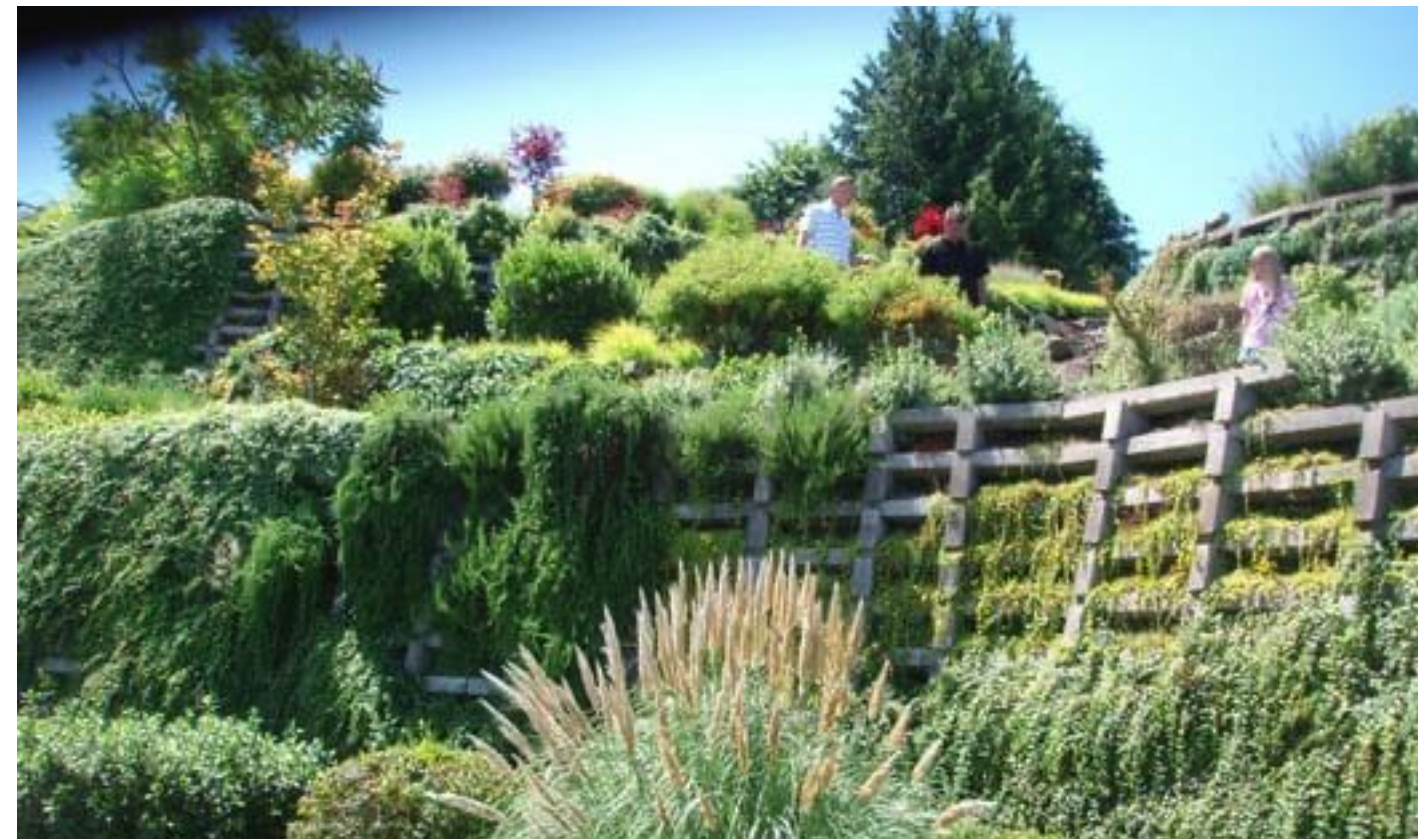
CRIBBLOCK RETAINING WALL
