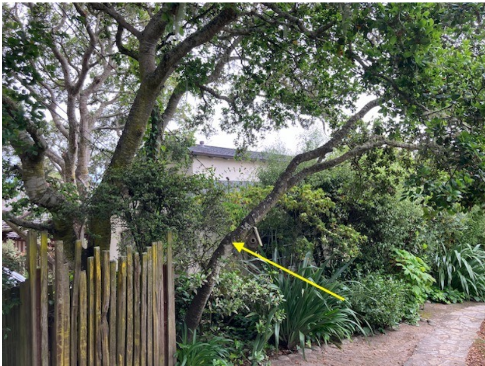
Figure 5. The small and suppressed oak identified as Tree#2 (yellow arrow) has a significant lean and poor structure and is proposed for removal due to construction impacts.
