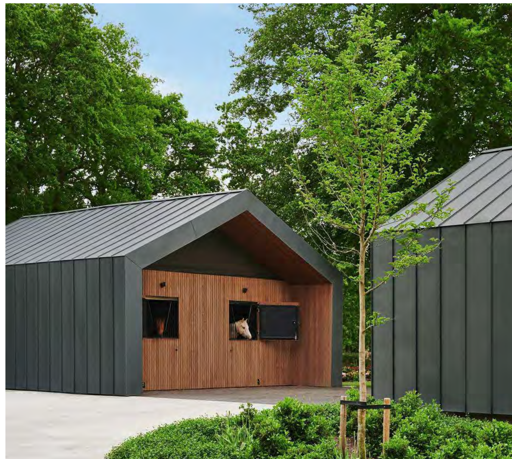
ROOF & FASCIA: RHEINZINK DOUBLE LOCK STANDING SEAM ROOF IN PRE-PATINA GRAPHITE GREY FINISH
