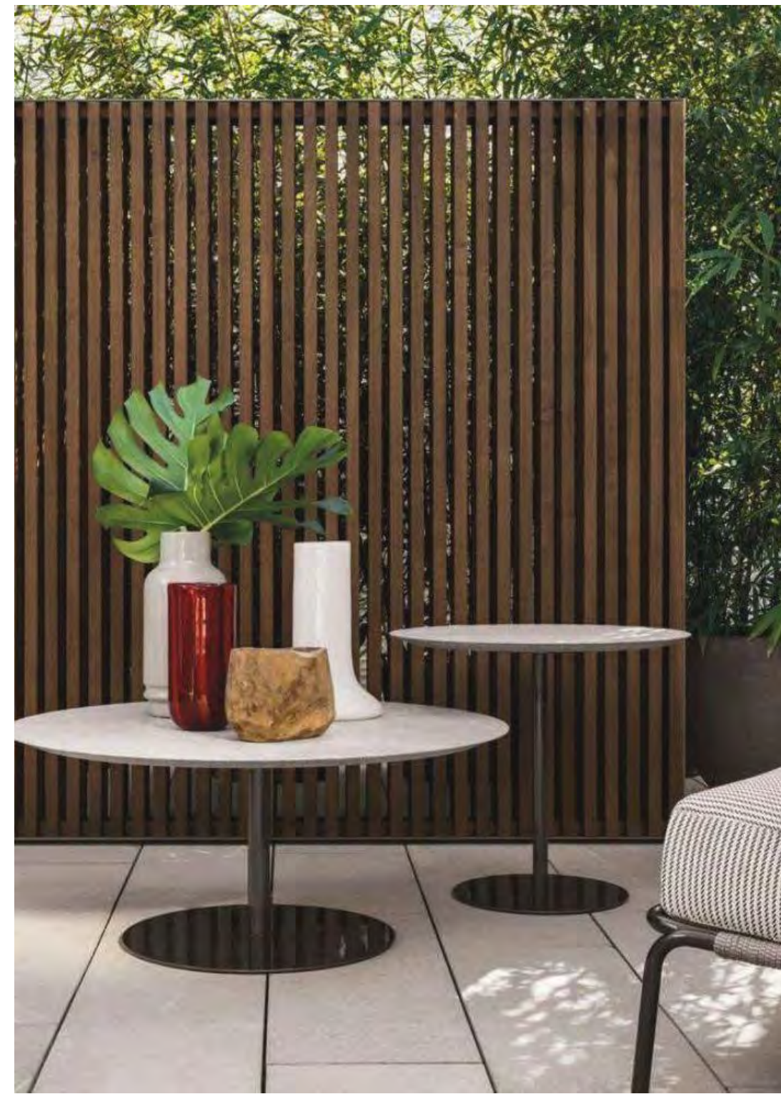
FENCING: 2x2 VERTICAL CEDAR SLATS SELF SPACED FINAL SPACING OF GAPS MAY VARY SLIGHTLY
