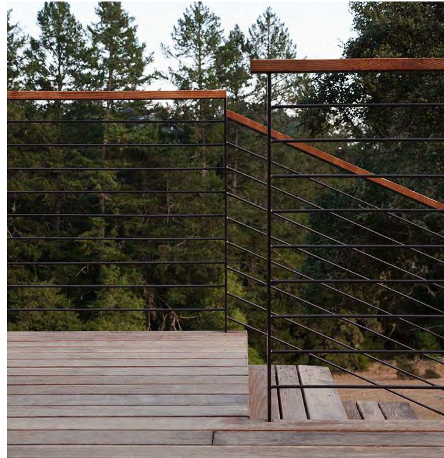
GUARDRAILS: POWDER COATED STEEL W/ IPE (WOOD) CAP. STAINED TO MATCH DECKING
