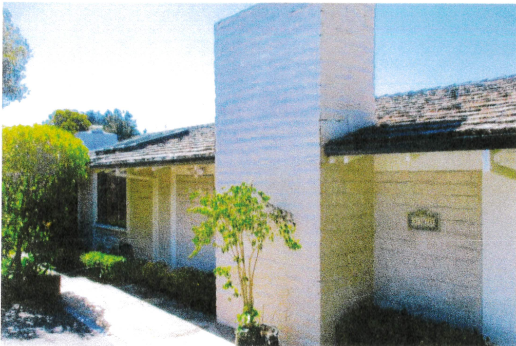
Photo #2, Looking SE at North facing facade, note c.1953 in fill of original garage for bedroom space, Kent Seavey, December, 2022.
