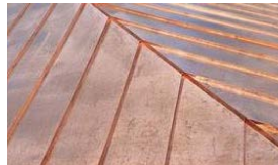
COPPER STANDING SEAM ROOM
