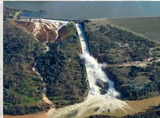
Photos of Oroville Spillway Failure 2017
