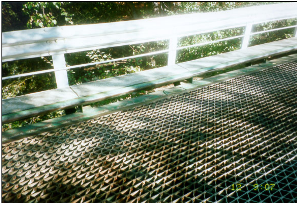
VIEW OF DECK STEEL GRATING
