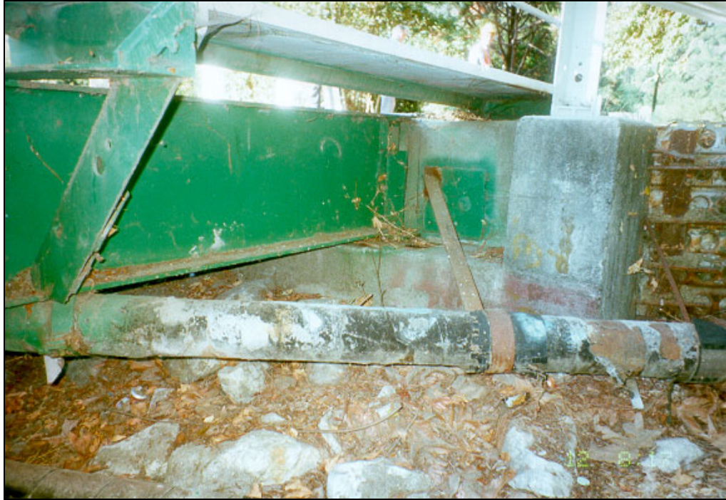
VIEW OF UTILITY PIPE AT SOUTH ABUTMENT
