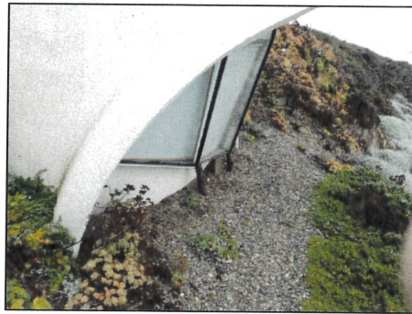
Plexi glass windows are leaking. Windows are failing. Makeshift support noted.
