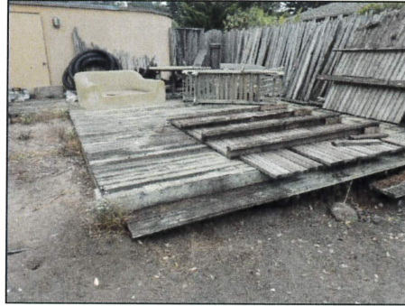
Deck found in poor condition.
