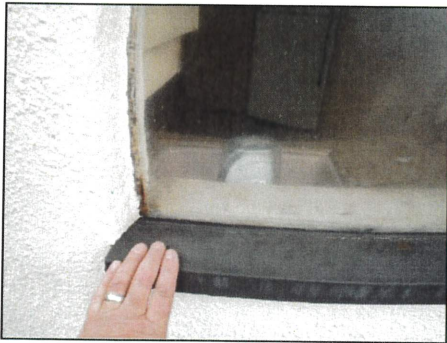
Plexi glass windows are leaking. Windows are failing. Makeshift support noted.
