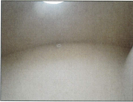
Some smoke detectors noted.
