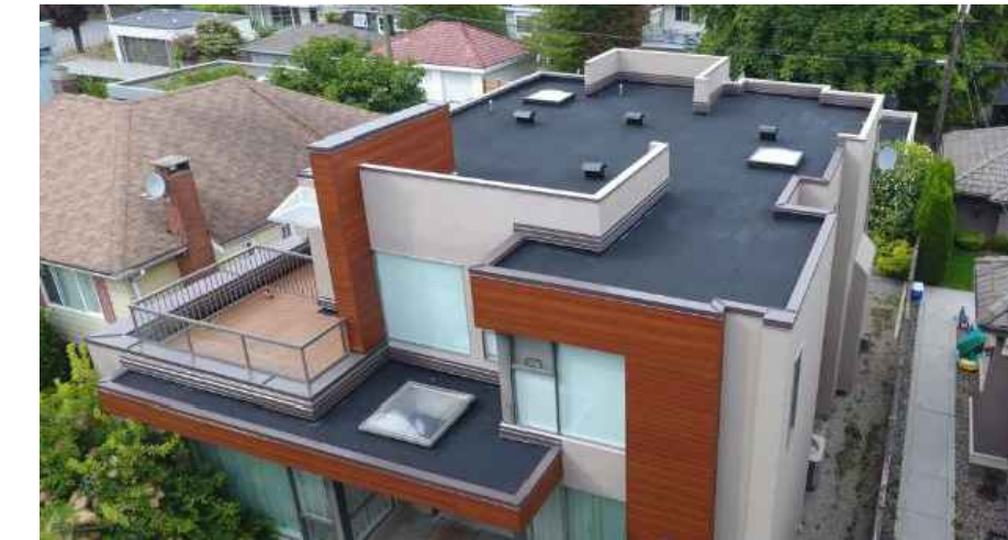
BUILT UP FLAT ROOF
