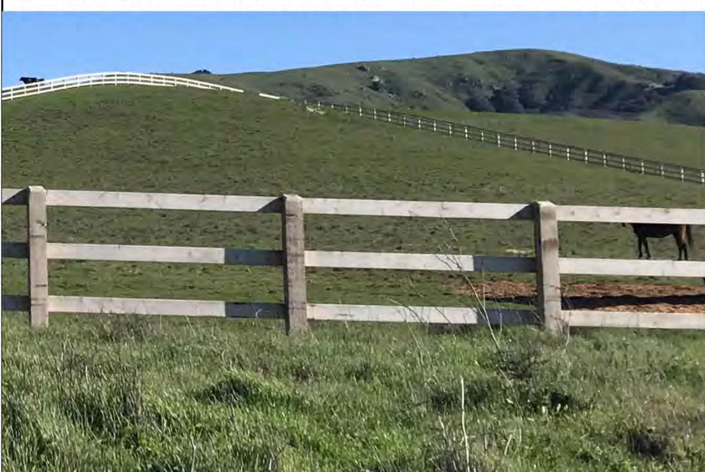
TYPE 3 HORSE PASTURE FENCE POST AND RAIL WOOD FENCE WITH MESH (DOG FENCE), 4'2" HT. SEE L4.02 DETAIL 6 NOTE: DRIVEWAY ACCESS, FENCES, AND GATE TYPE AND LOCATION PENDING DISCUSSION WITH THE CONSERVANCY AND THE OWNER.
