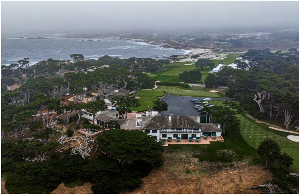
Photograph No. 2: Overview of Clubhouse Building, Garage, and Pro Shop/Candidate Building, Portions of Golf Course Included, View Northeast
