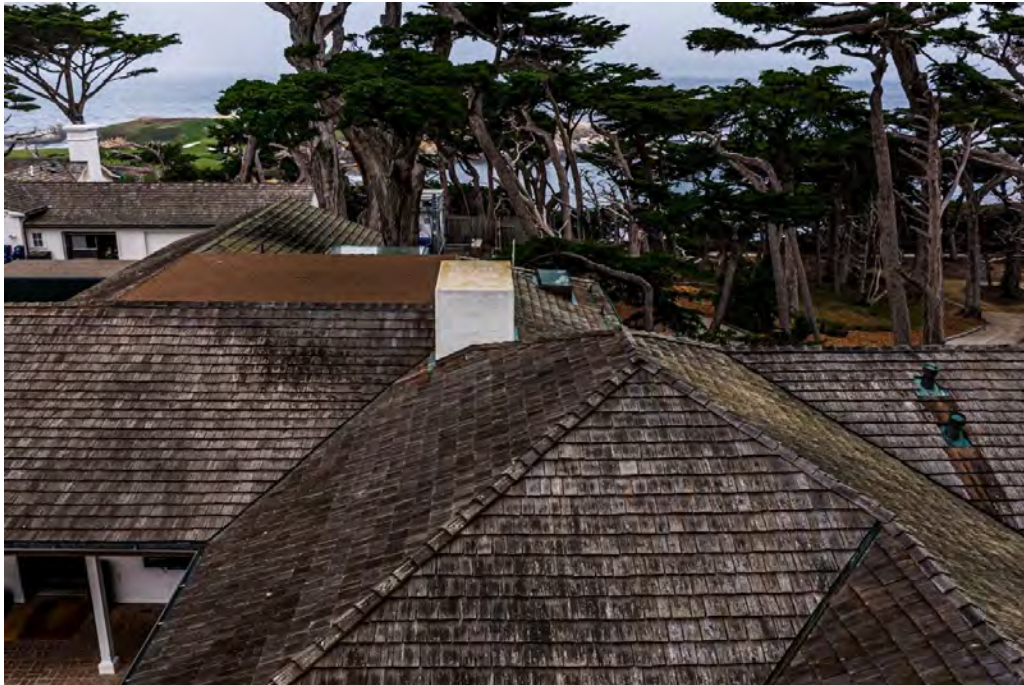
Photograph No. 6: Close-up view of roof area of Pro Shop/Candidate building Faux Chimney structure location, View West
