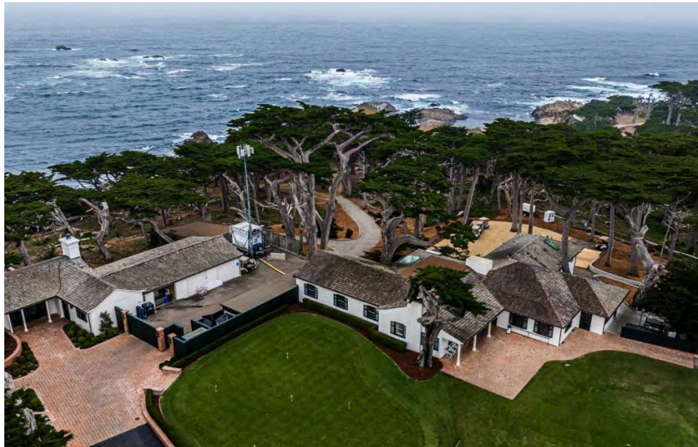
Photograph No. 4: View of Cypress Point Club Pro Shop/Candidate Building, East and South Elevations, Candidate Location is to the right in the photo. Garage is in rear of Pro Shop building. A temporary Cell on Wheels (COW) is evident to the center left of photo; Garage is located behind Pro Shop Building left of Cell Tower Equipment; View Northwest
