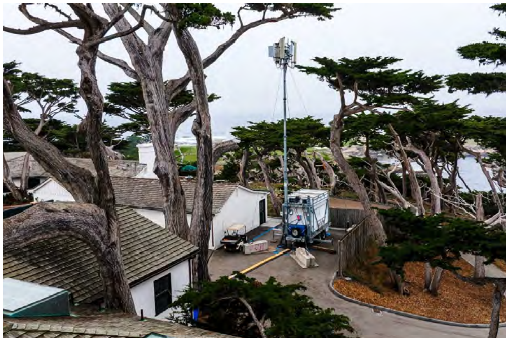
Photograph No. 5: View of Cell on Wheels (COW) currently located behind Pro Shop/Candidate building, Garage is located behind Pro Shop building and to the left side of the cell tower equipment; View West
