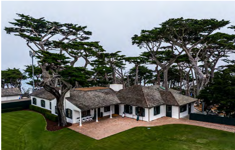
Photograph No. 3: View of Pro Shop/Candidate Building, East and South Elevations, Candidate Location is Faux Chimney Structure in Center of Roof Area, View Northwest
