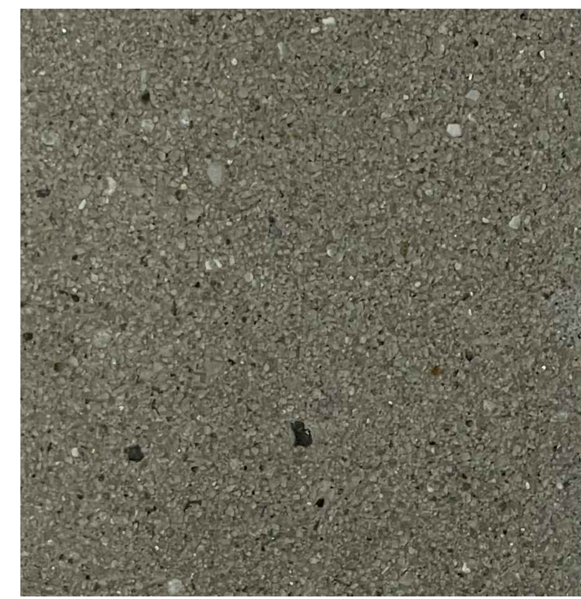
8 CHIP SEAL PAVING
