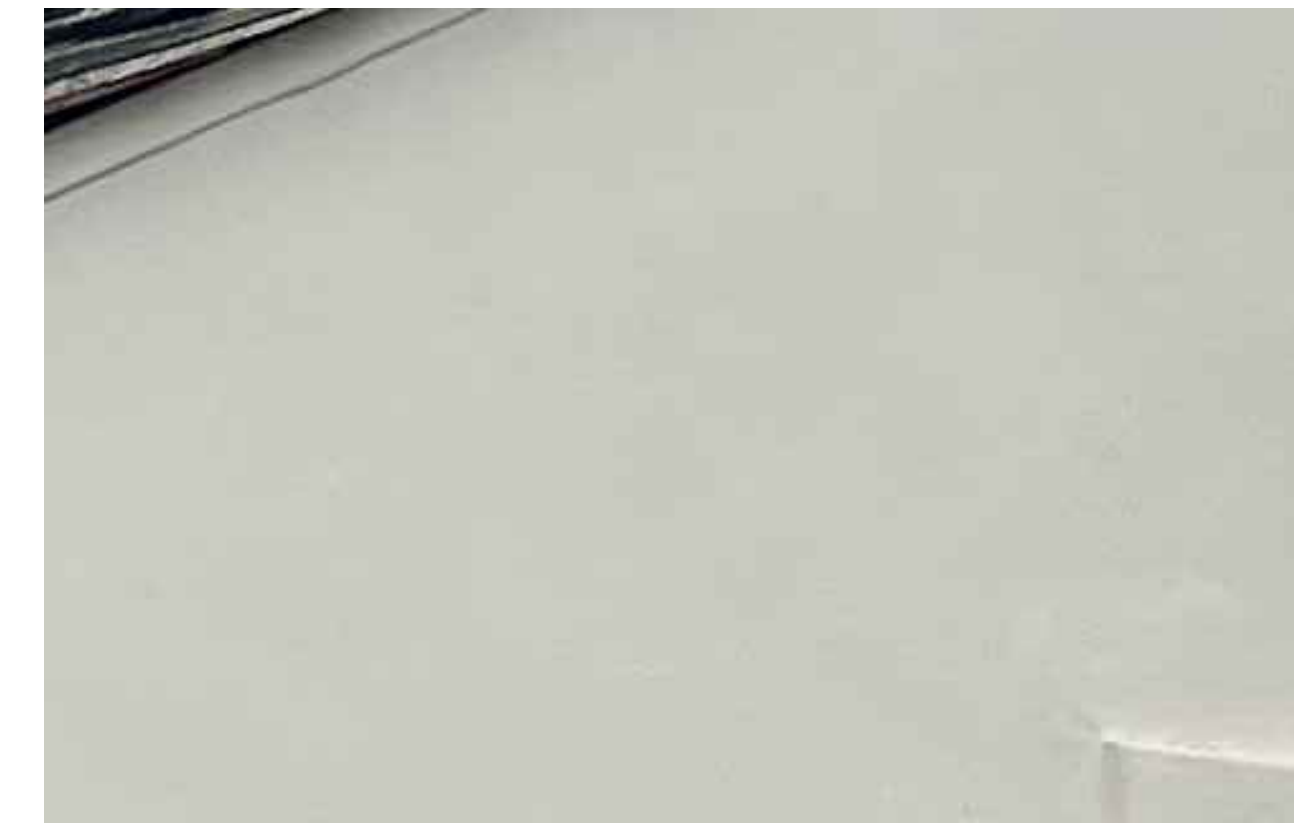
A NEW CEMENT PLASTER SIDING COLOR TO MATCH EXISTING
