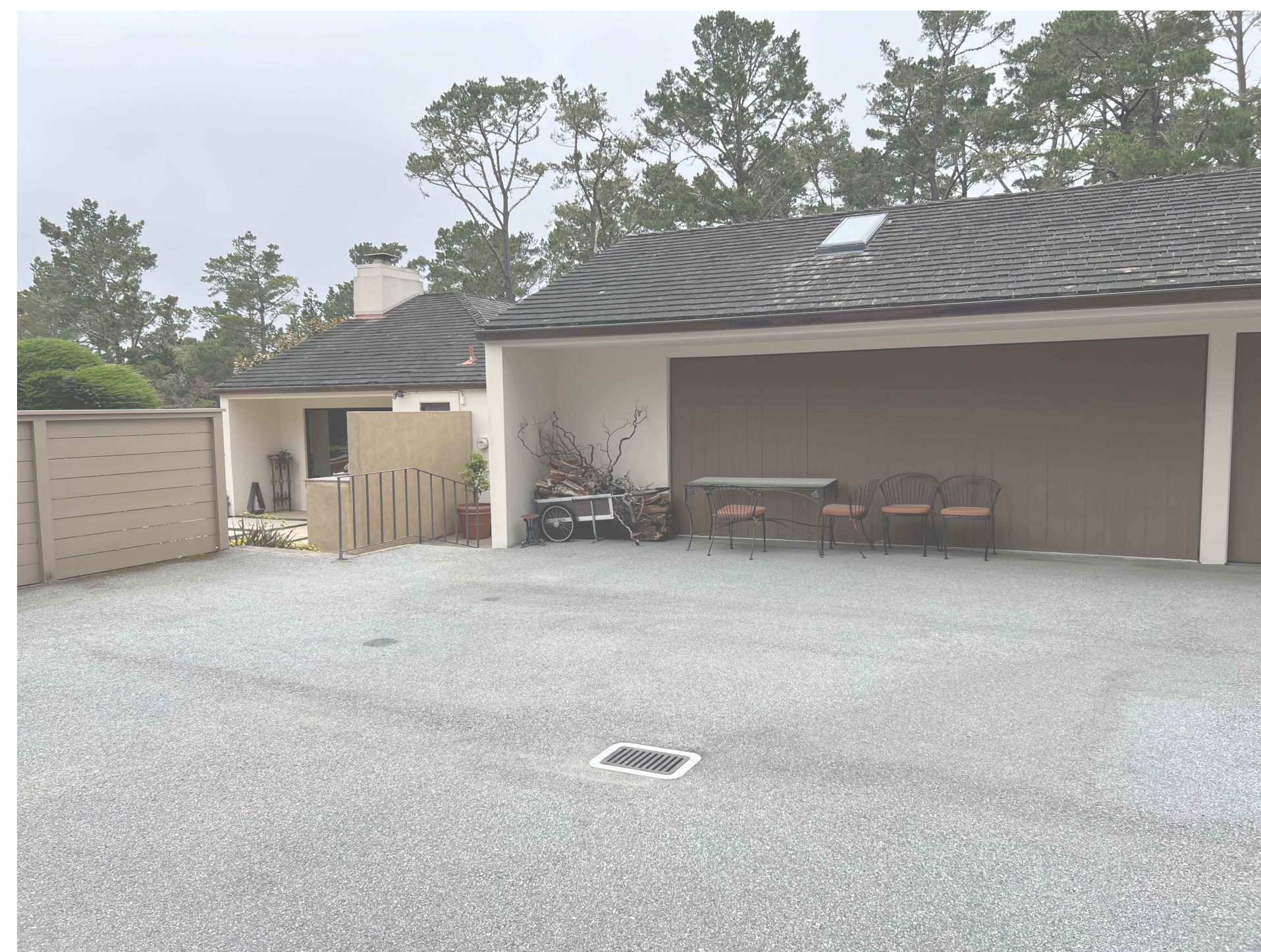
2 EXISTING PHOTOGRAPH LOOKING WEST AT EXISTING GARAGE & EXTERIOR SIDE OF KITCHEN TO BE RENOVATED WITH NEW ADDITION
