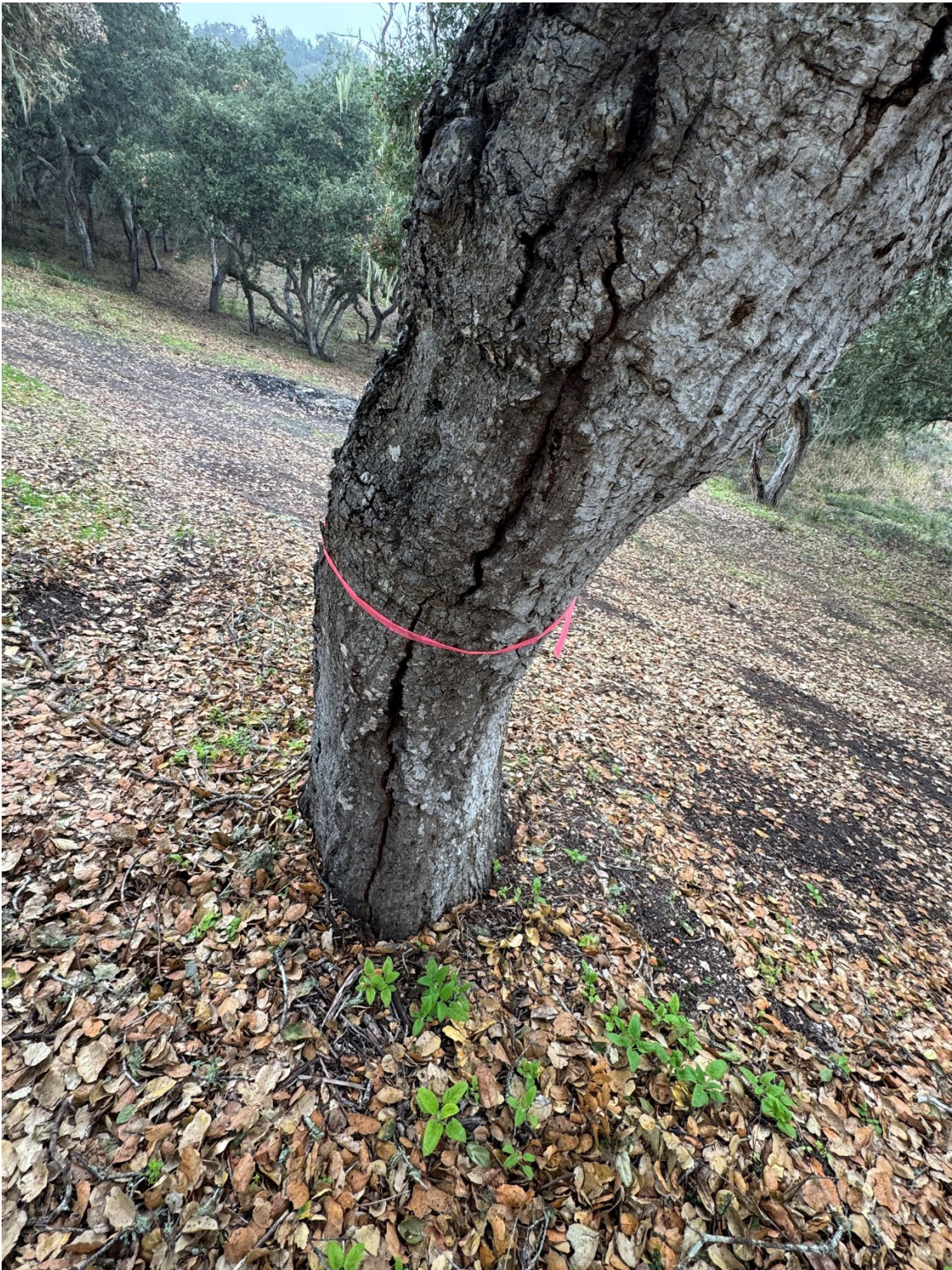
Fractured stem on the compression side of the trunk
