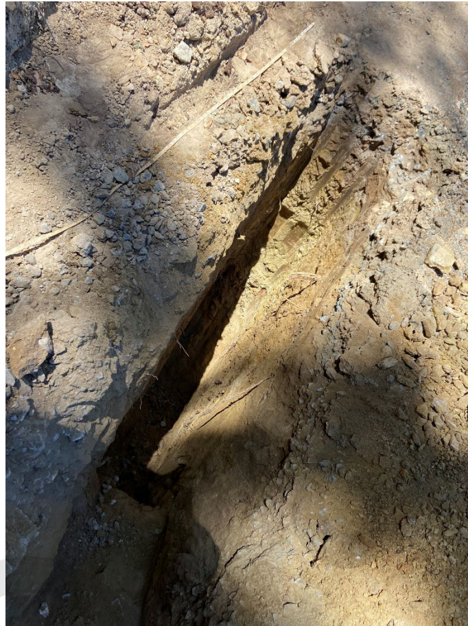
Photo #4: Excavation of TP-2, Downhole
