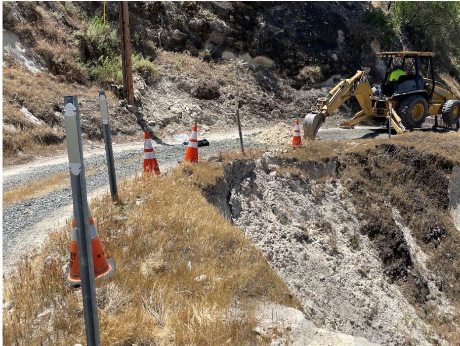
Photo #5: Excavation of TP-3, Looking West
