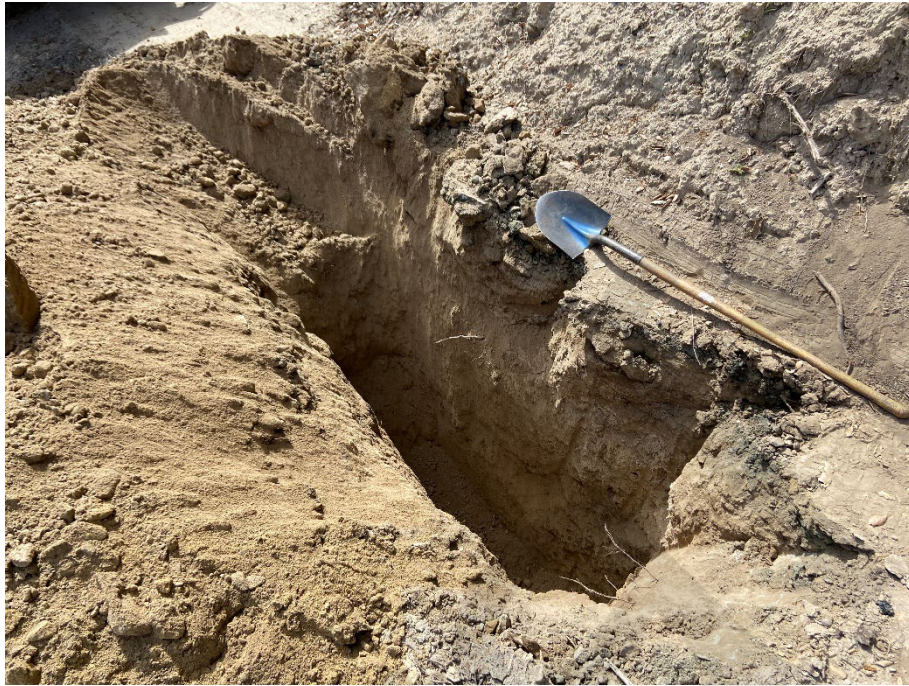
Photo #3: Excavation of TP-1, Artificial Fill Zone
