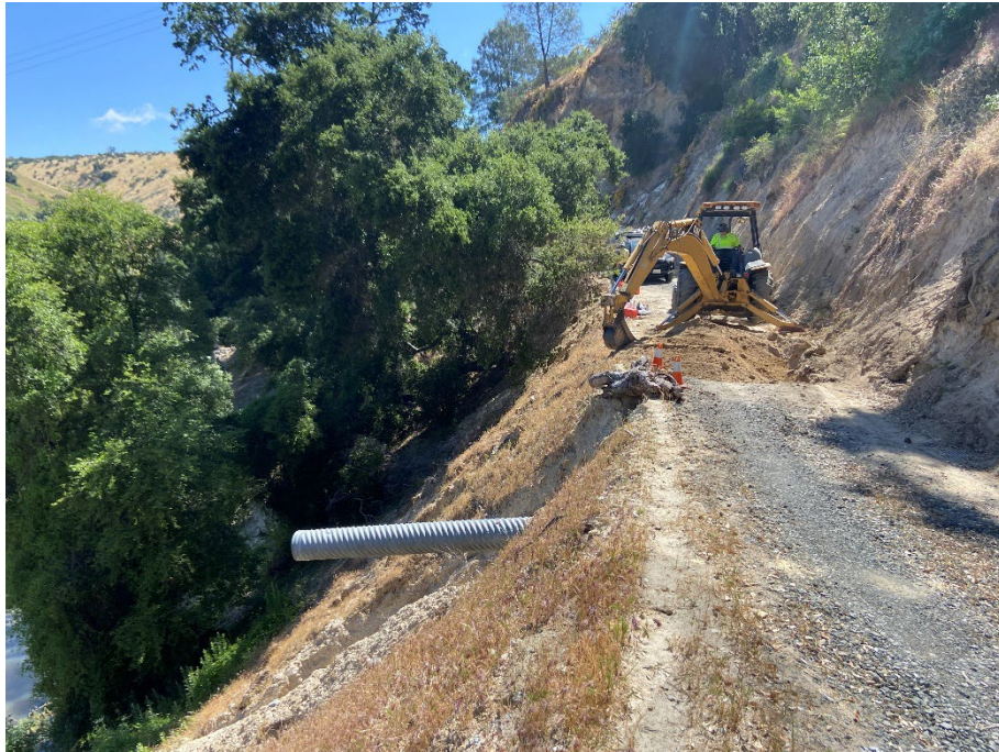
Photo #1: Excavation of TP-1, Looking East
