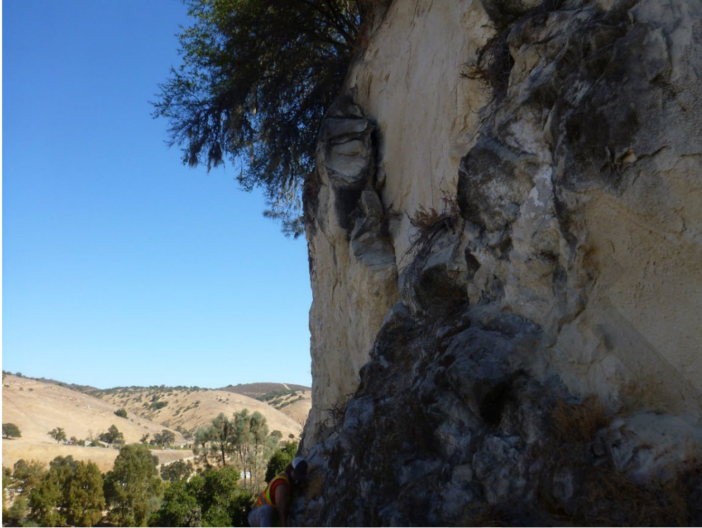
2019 Photograph 5. Rock cut for access road above Powerhouse. Note roots behind slab of sandstone.
