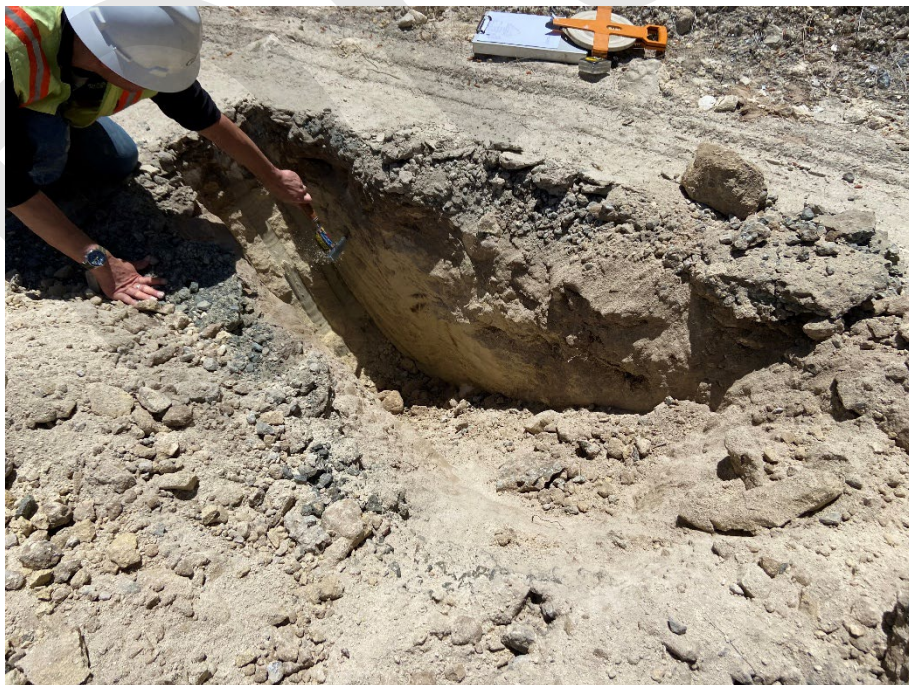
Photo #6: Excavation of TP-3, Downhole
