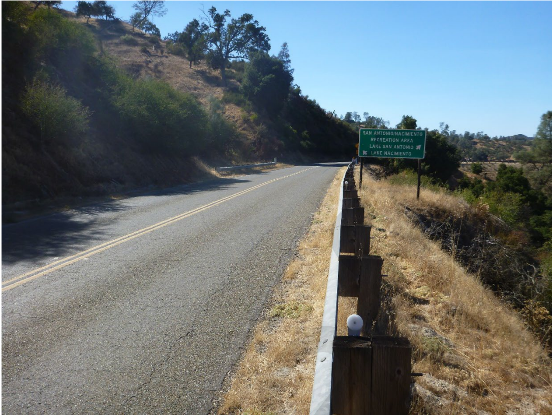
2019 Photograph 12. General condition of roadway, showing minor cracks.
