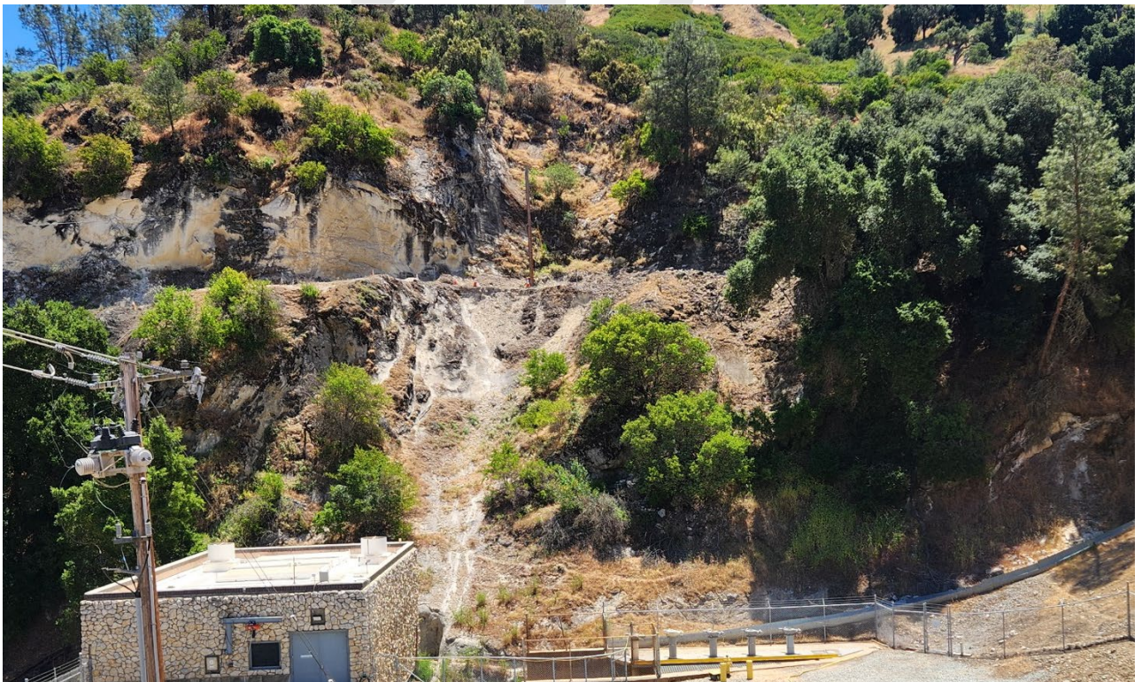
2024 Photograph 1. Minimal change from 2019. Arrow indicates minor slump within swale.
