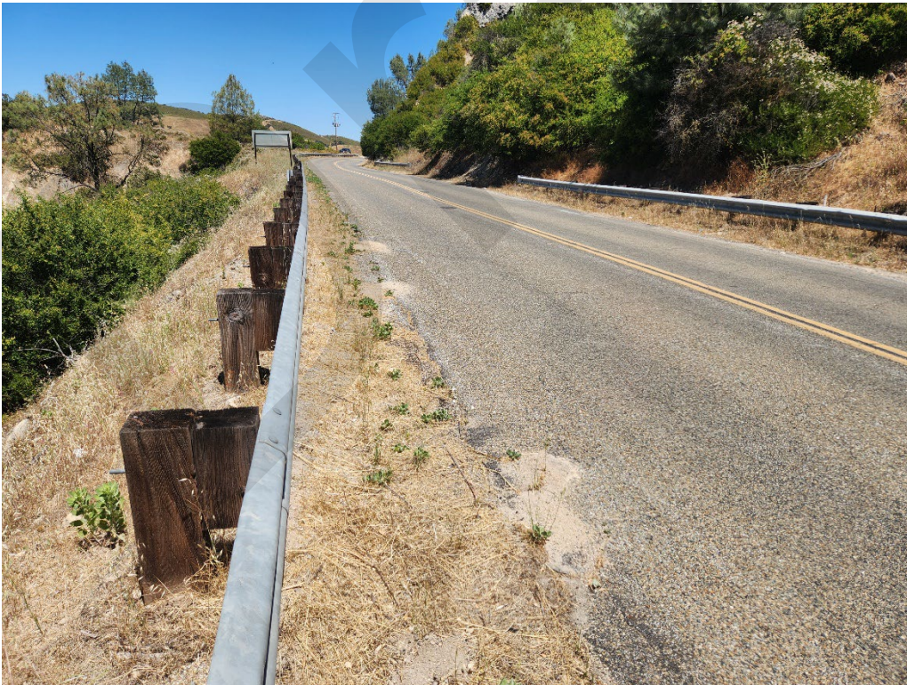
2024 Photograph 16. No discernable change from 2019.
