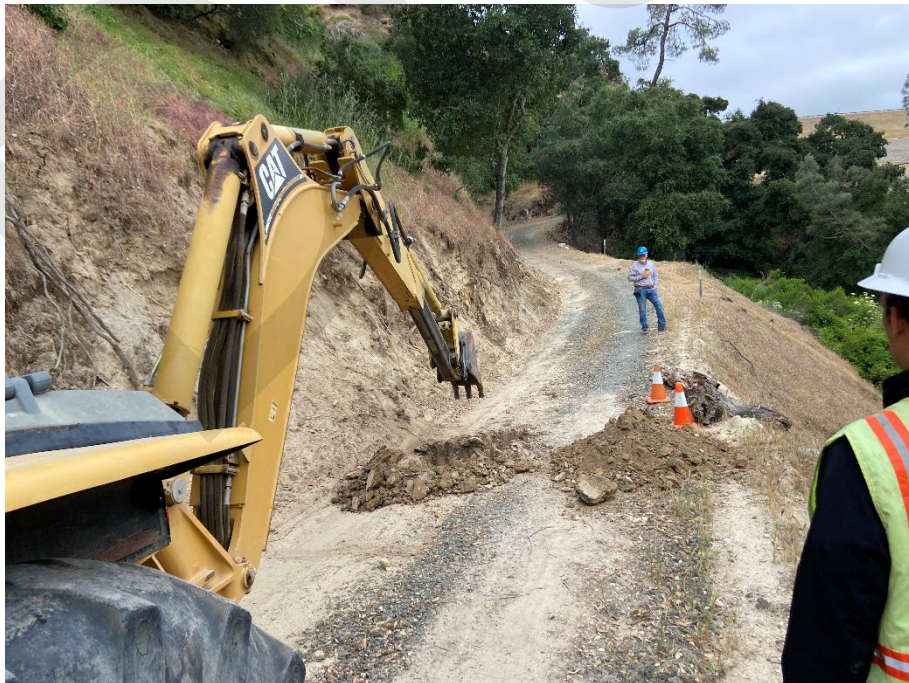
Photo #2: Excavation of TP-1, Looking West
