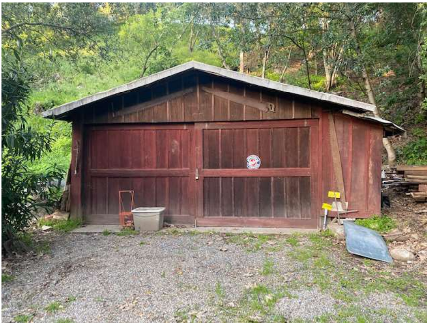
Existing Garage to be Demolished
