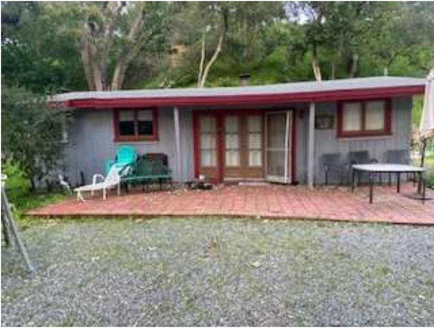
Existing House to be Demolished
