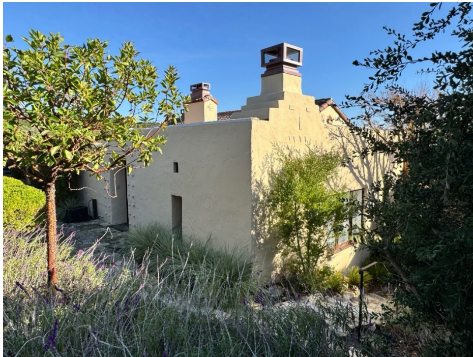
Figure 9. North and west elevations, facing southeast.
