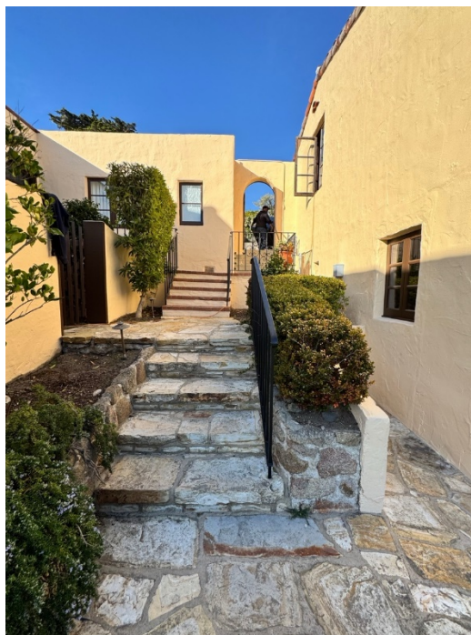
Figure 29. South elevation of east wing, with wing wall connected the 1920 house to ca. 1930 garage, facing north.
