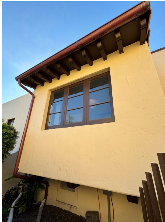
Figure 28. Projecting bay window on the east elevation, facing southwest.
