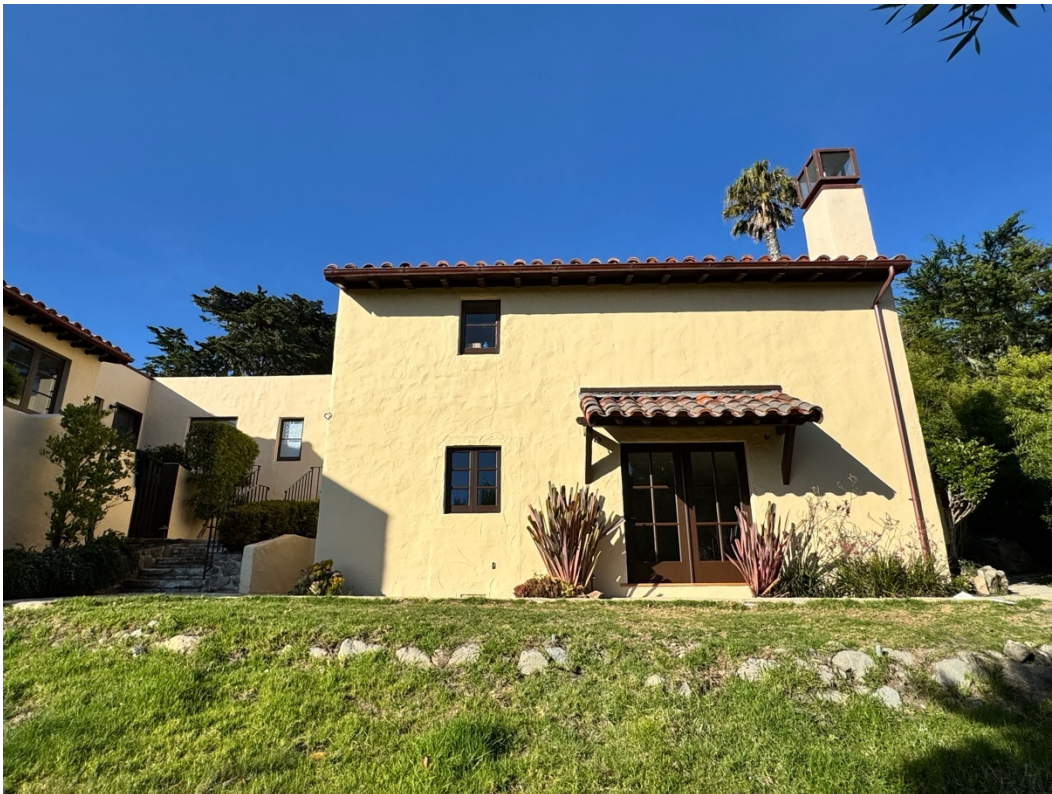
Figure 37. South elevation, facing north.
