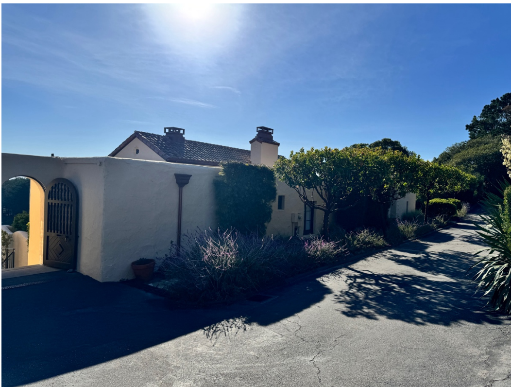
Figure 1. North elevation, facing southwest.
