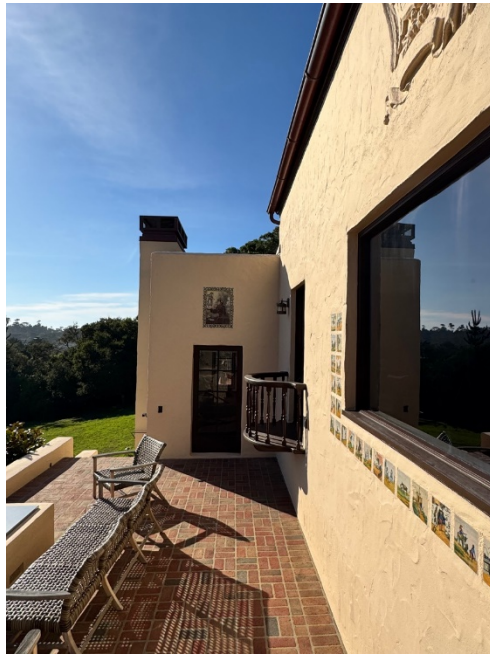
Figure 15. East wall within raised patio, with single wood door and tile portrait of St. Anthony of Padua.
