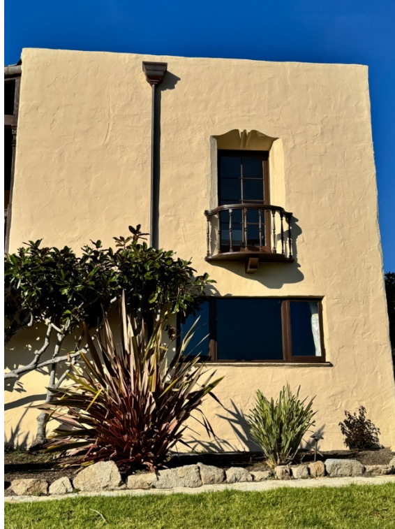
Figure 43. Eight-light wood door set within decorative alcove with Juliet balcony above picture window, facing north.
