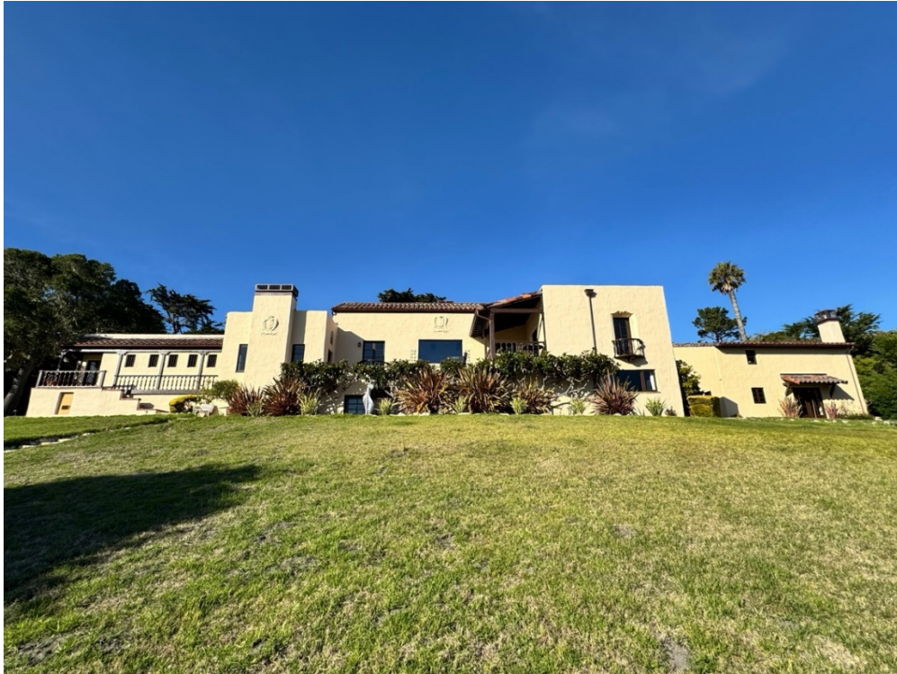
Figure 17. South elevation, facing north.
