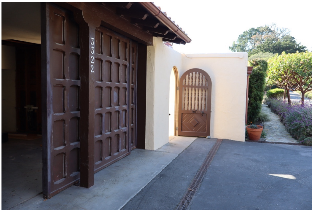
Figure 40. Arched gate through wing wall.
