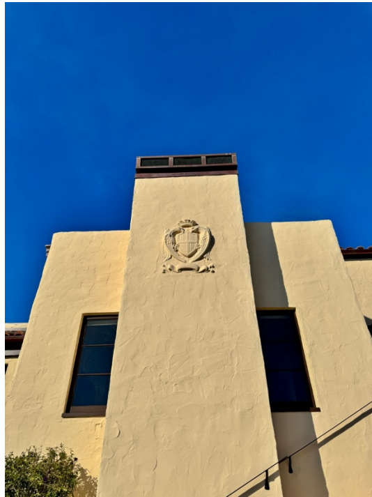
Figure 21. Exterior stucco chimney on south elevation, facing north.
