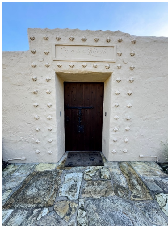
Figure 5. Entrance to loggia and courtyard, facing south.
