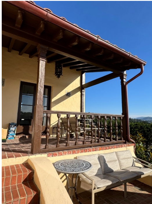
Figure 26. Raised covered porch.
