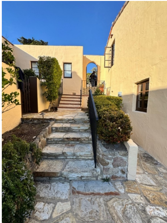
Figure 44. South elevation of east wing, with wing wall connected the 1920 house to ca. 1930 garage, facing north.
