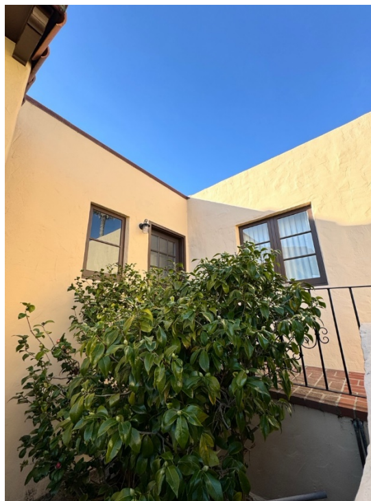
Figure 14. Two-light fixed wood windows and a single wood window, facing northwest.
