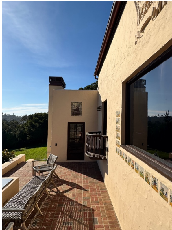
Figure 30. East wall within raised patio, with single wood door and tile portrait of St. Anthony of Padua.
