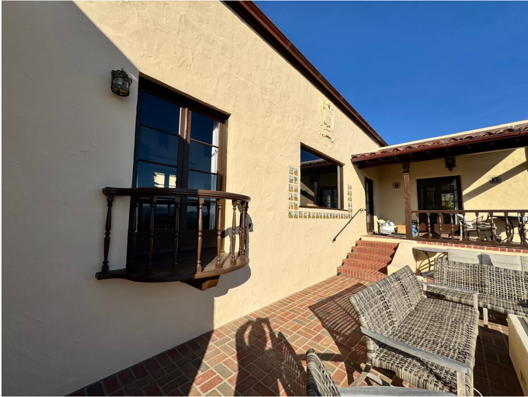
Figure 39. South elevation within the raised patio, facing northeast.
