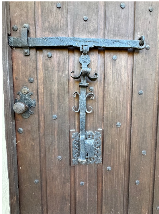
Figure 23. Wood door with hand-forged wrought iron details, bolt, key hole and door knob, with “G T C” carved into the iron trim plate.
