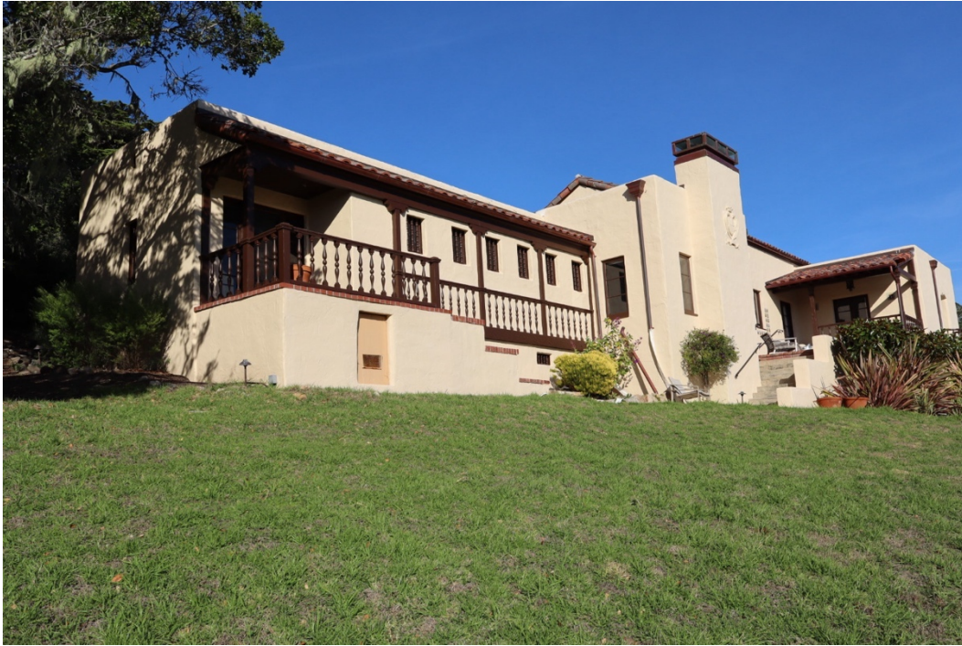
Figure 33. South and west elevations, facing northeast.
