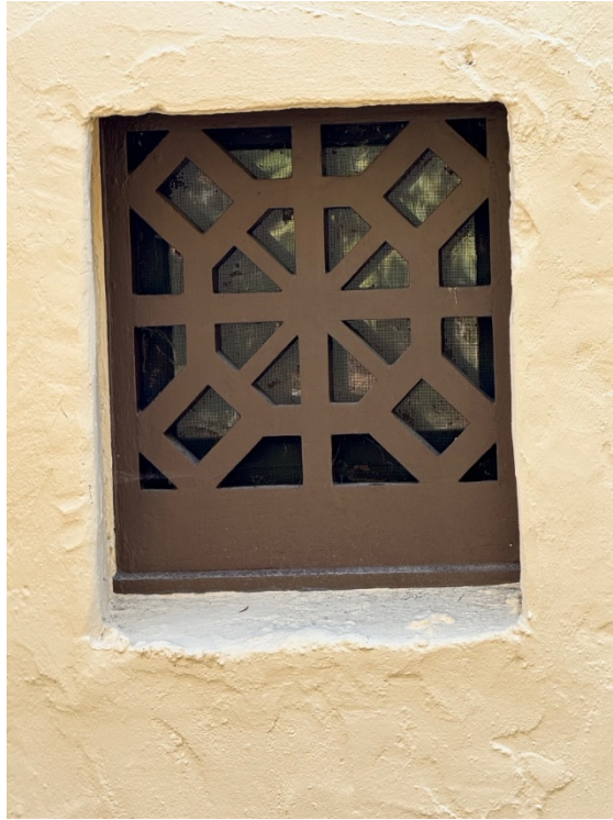
Figure 18. Detail of geometric wood grille.
