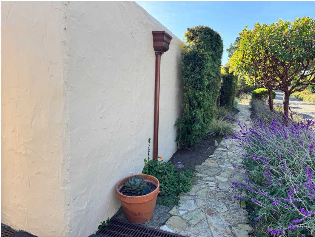
Figure 17. East wing of north elevation, facing southwest.
