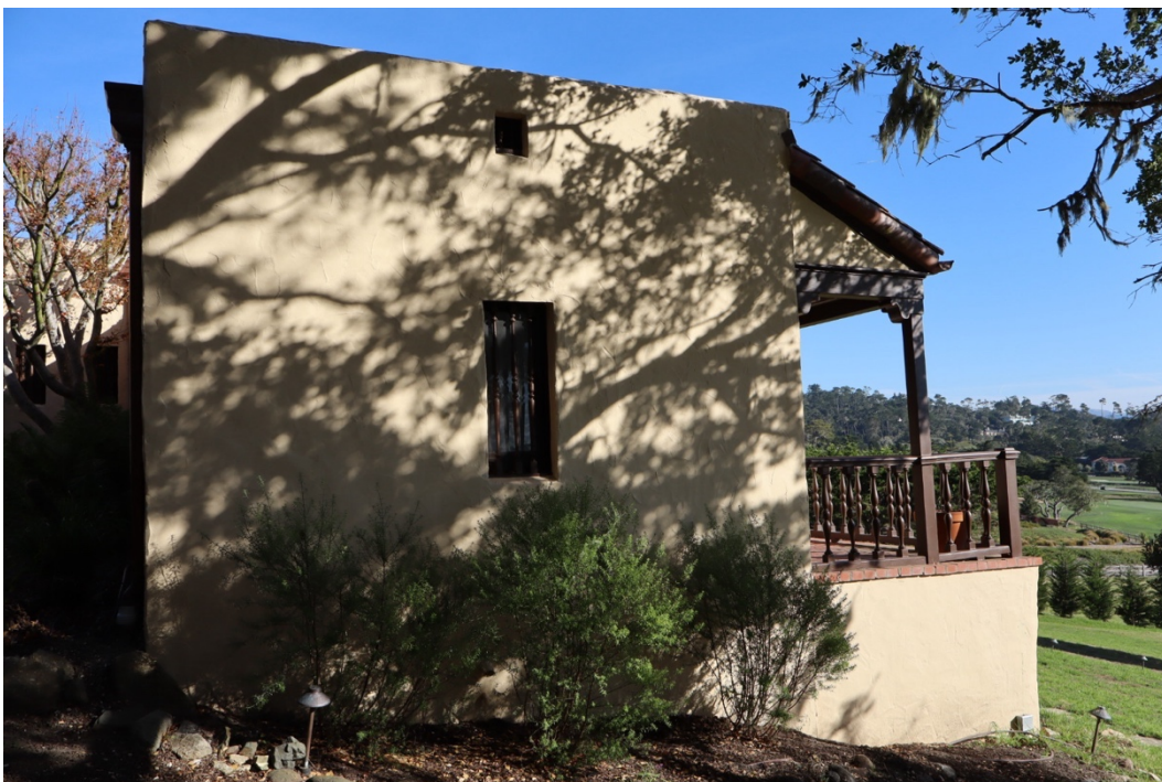
Figure 32. West elevation of west wing, facing east.
