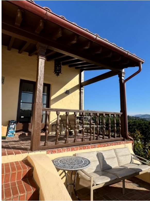
Figure 41. Raised covered porch.
