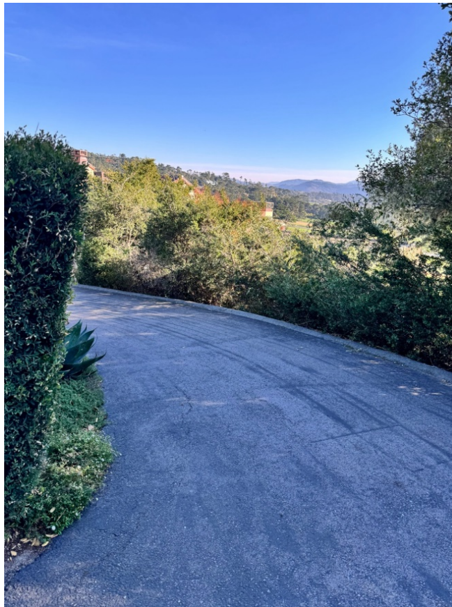
Figure 53. Entrance to the driveway of 1920 house.
