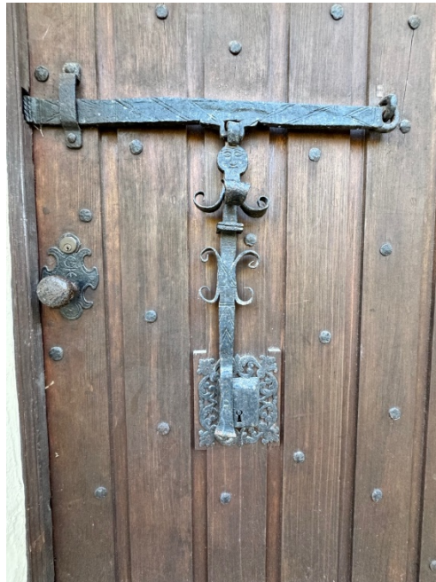
Figure 8. Wood door with hand-forged wrought iron details, bolt, key hole and door knob, with "G T C" carved into the iron trim plate.
