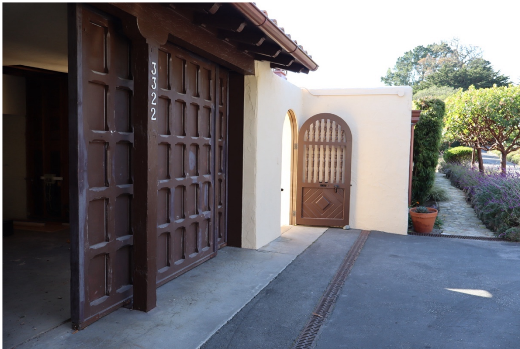
Figure 55. Arched gate through wing wall.
