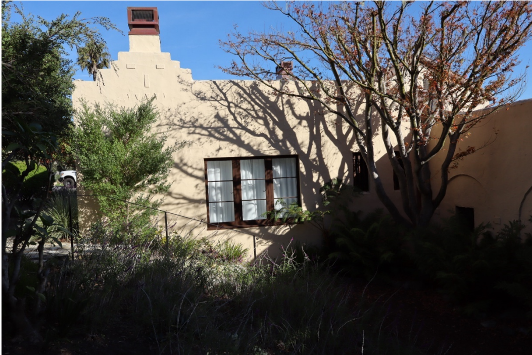
Figure 31. West elevation with stepped parapet to stucco chimney, facing east.
