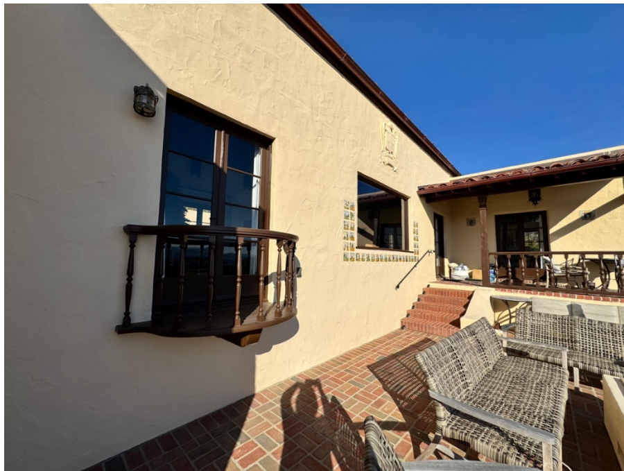
Figure 24. South elevation within the raised patio, facing northeast.
