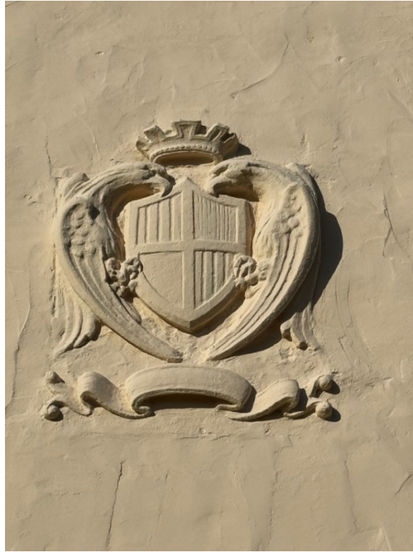
Figure 37. Stucco cartouche on exterior stucco chimney of the south elevation.
