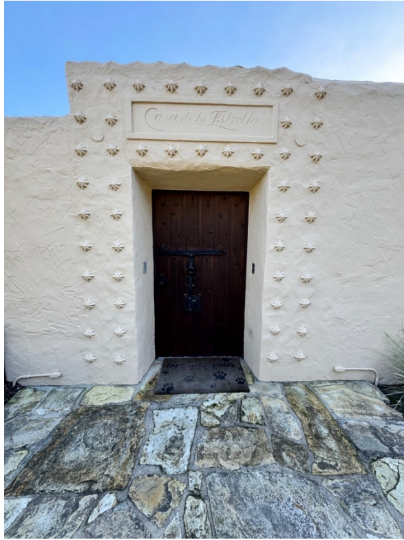
Figure 20. Entrance to loggia and courtyard, facing south.
