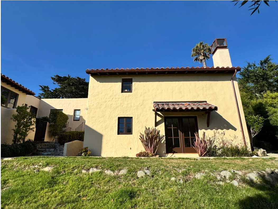
Figure 52. South elevation, facing north.
