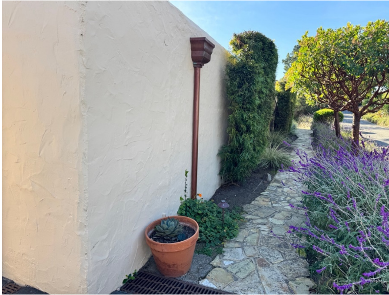
Figure 2. East wing of north elevation, facing southwest.
