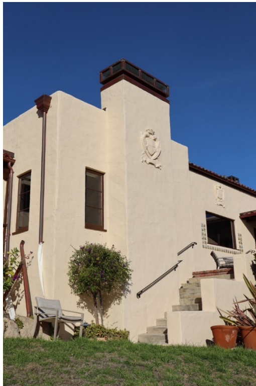
Figure 20. Exterior stucco chimney and steps leading to rear, raised patio, facing northeast.
