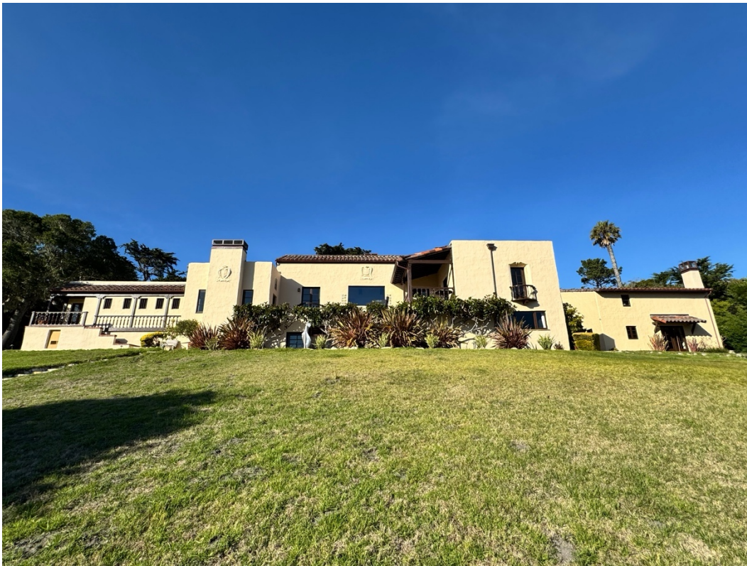
Figure 32. South elevation, facing north.
