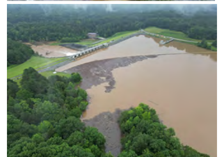
Spillway Gate Protection
