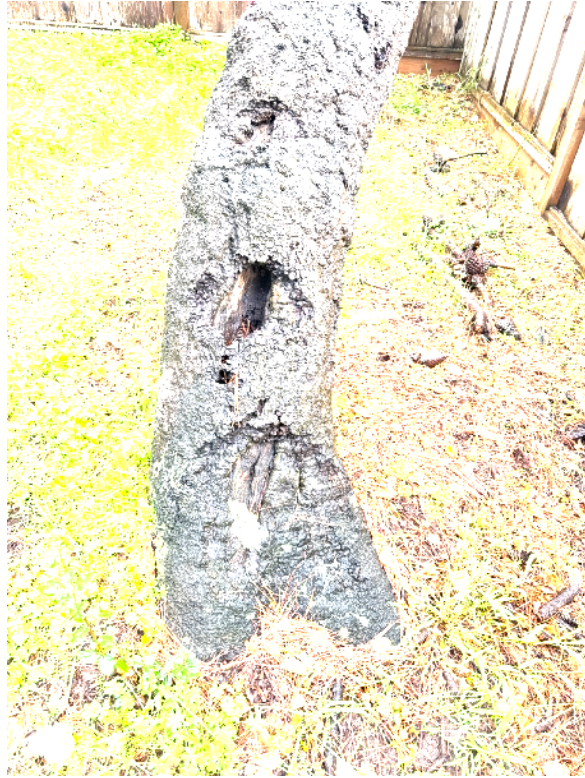
Subject tree 891 - Is in decline with advanced decay and cavities. The canopy develops beyond the critical root zone increasing the likelihood of failure.
