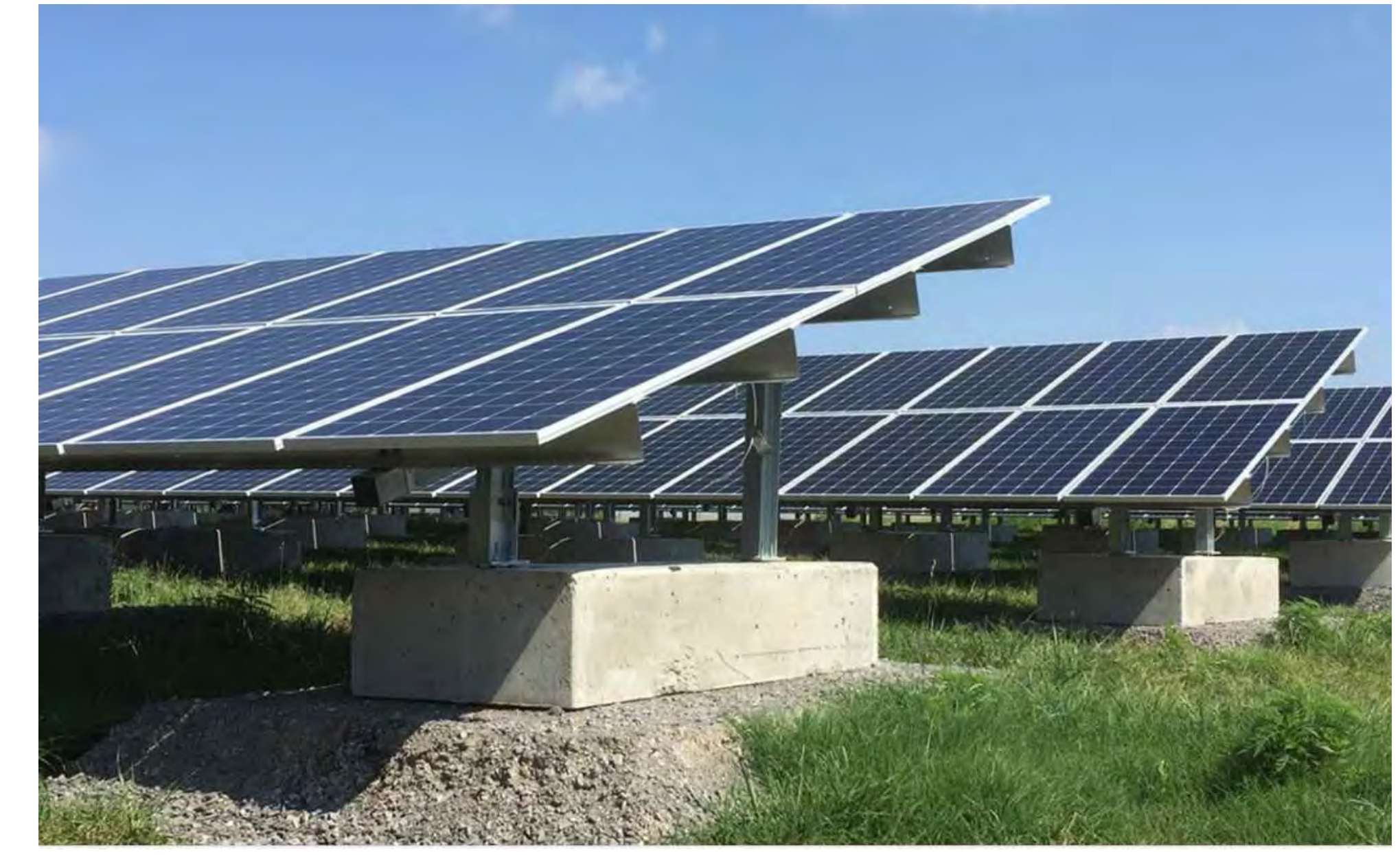
TYPICAL FIXED TILT RACKING ON BALLASTED FOUNDATIONS
