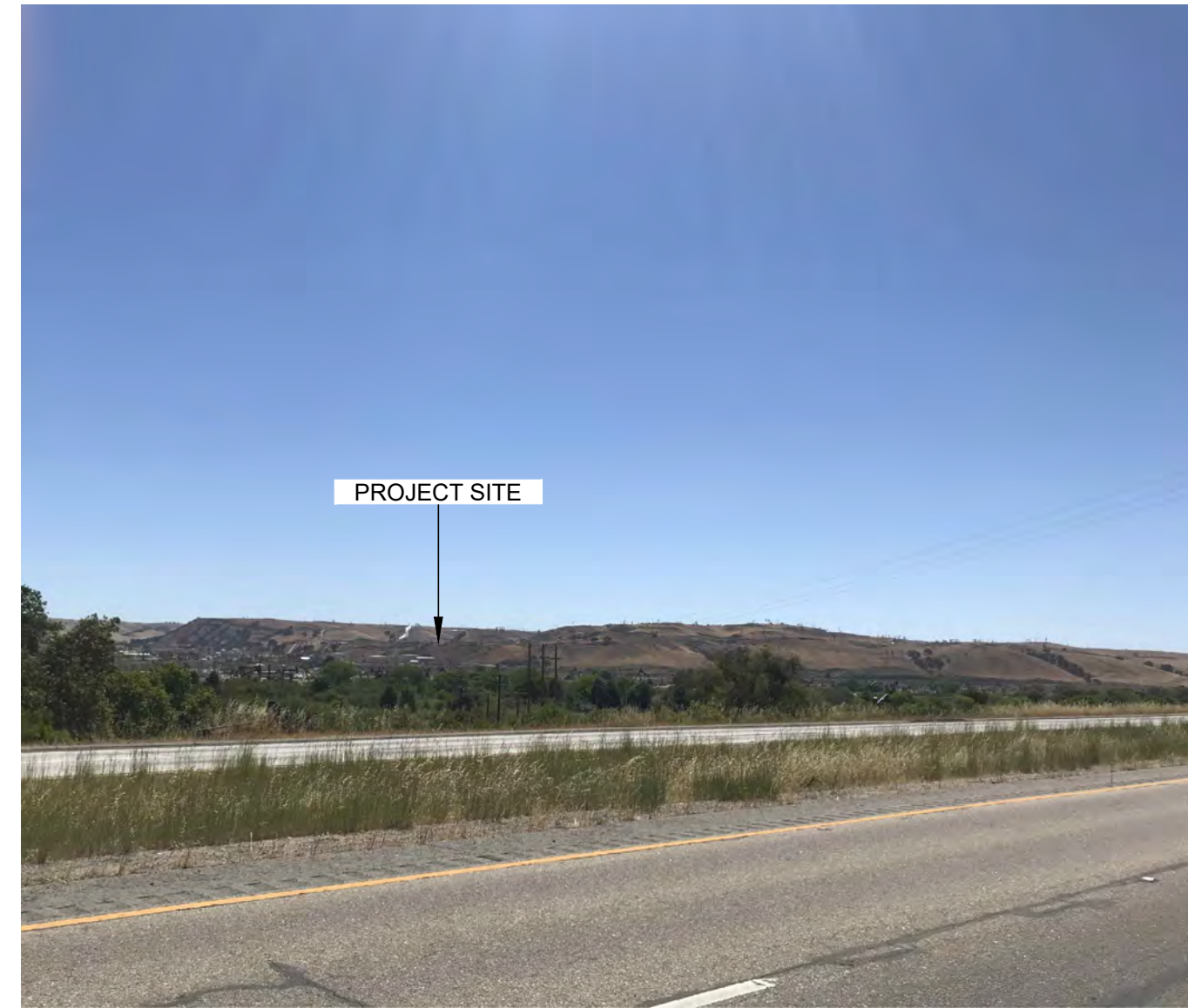
2 VIEW FROM SOUTHBOUND HWY 101
