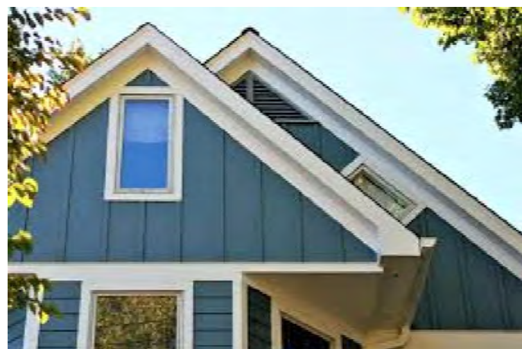
1 HARDIEPANEL VERTICAL SIDING: CEDARMILL - BOARD-AND-BATTEN SCALE: NTS
