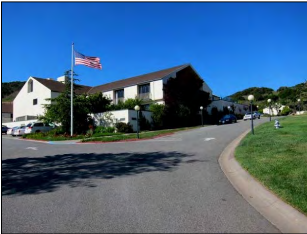
Figure 2. Looking northeast toward Pavilion Building.
