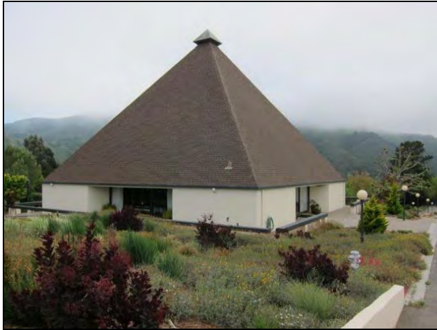
Figure 21. Side (east) elevation of Meeting House.
