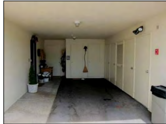
Figure 36. Typical garage design seen on Bldg. 22.
