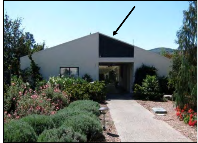
Figure 26. Rear (north) elevation of the West Parlor. Connection of two shed roofs shown with an arrow.
