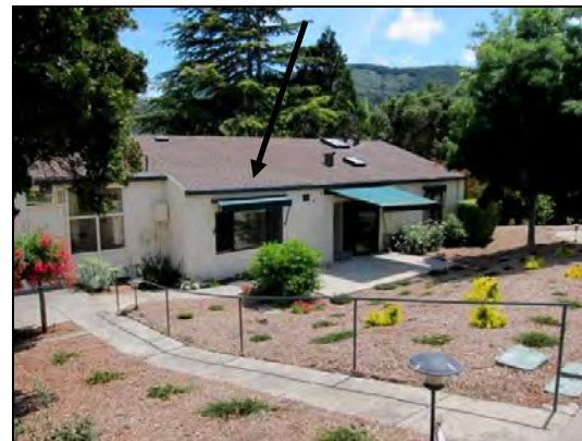
Figure 38. Rear of Bldg. 29 showing garage conversion.
