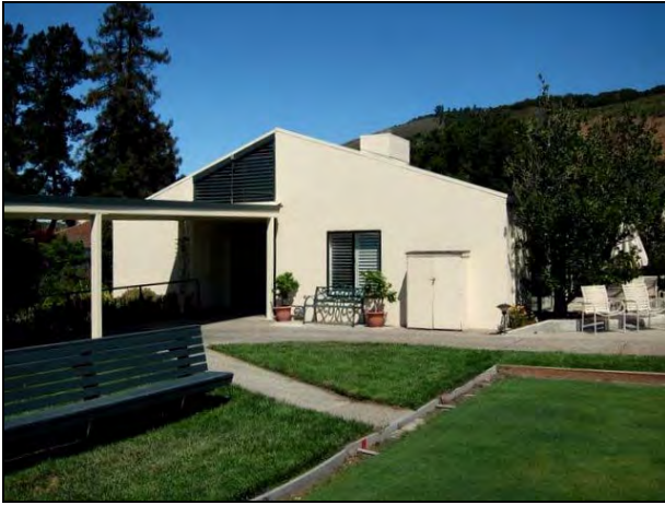
Figure 25. Front (south) elevation of the West Parlor. Note the covered walk leading to the façade.
