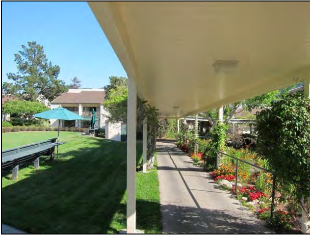
Figure 10. Covered walk leading to Pavilion Building.
