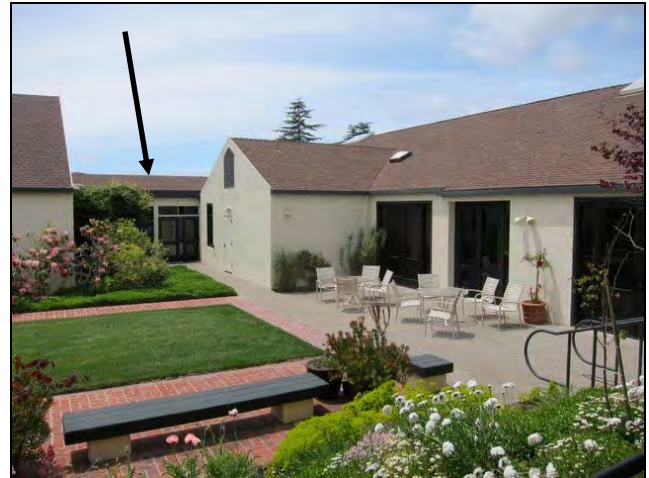
Figure 20. The highly-modified Infirmary, now the Resident Activity Center. Arrow indicates the connecting structure.
