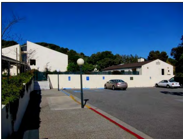
Figure 4. Looking east toward Bldg. 17 and Fitness Center from main parking lot.
