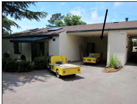
Figure 37. Bldg 29 conversion of garage to study.
