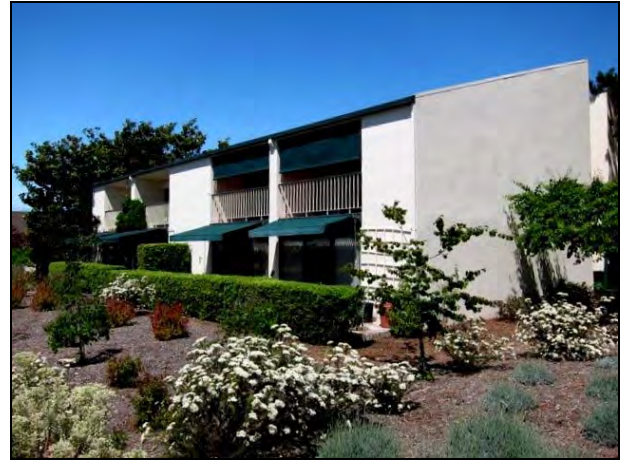
Figure 28. Side (north) elevation of Bldg. 14.
